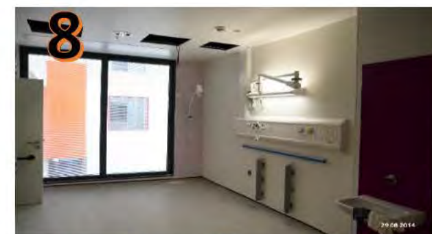
Typical Ward 2b Ensuite Bedroom (29 Aug 14)
