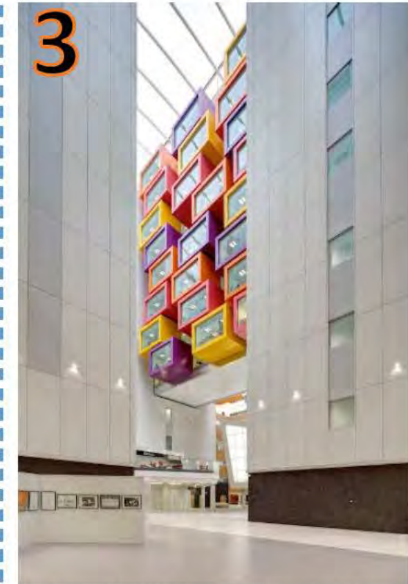
3 View of link bridge from Imaging Dept (28 April 2015)
