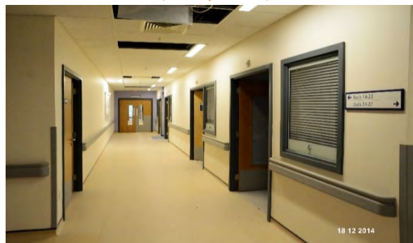
Typical view towards corner of ward leg (18 Dec 14)
