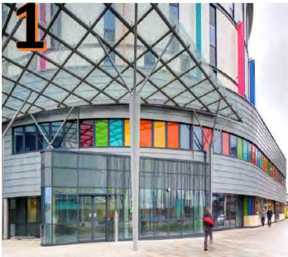
1 Main Entrance – NCH (26 Aug 15)
