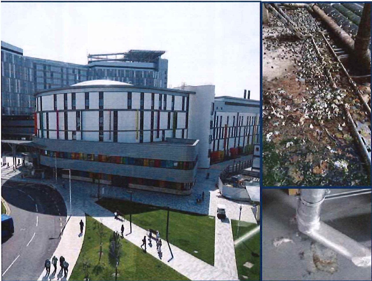
Outstanding repairs and the discovery of bird droppings have heightened infection fears at QEUB
