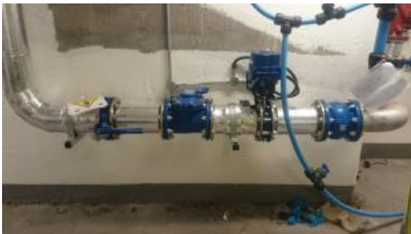
Hardgate Road mains including temporary supply for commissioning
