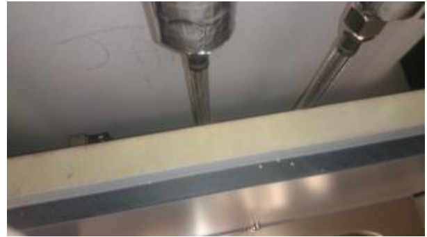
EPDM flexible hoses fitted at double level sinks in facilities room (DSR's)
