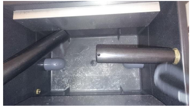
Dental CWST (Empty at time of survey)
