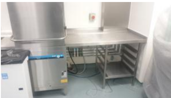
EPDM flexible hose to dishwashers
