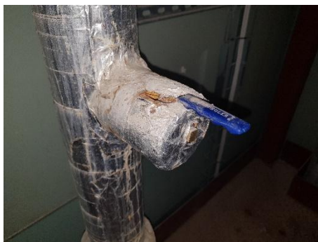
CA8-006 Injection Valve Open
