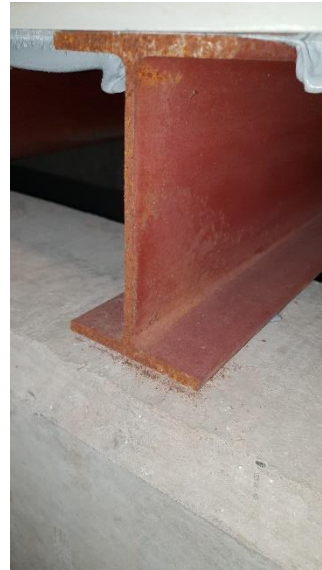
Example – non galvanised CWST steel supports
