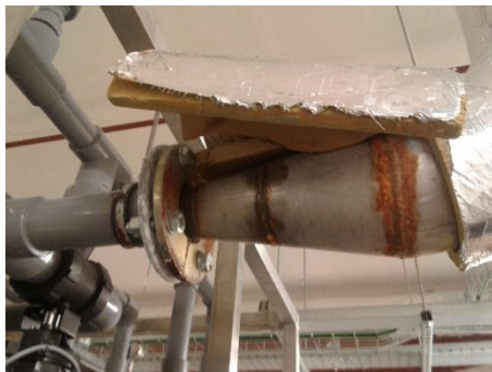
Basement Leaking Flange at Filter Unit
