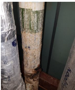
GENW11-068 Evidence of Leak
