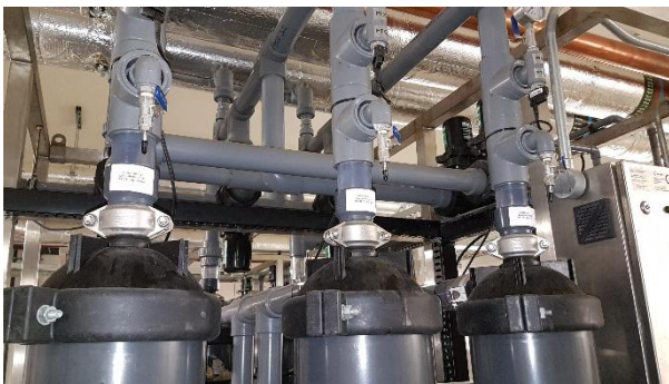
Filter with Sample Point Caps
