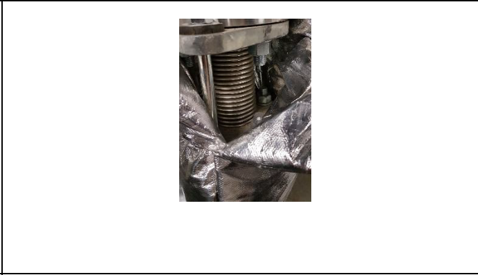
P41 Cal Return Pump Coupling
