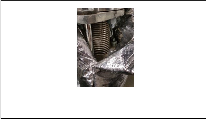
P41 Cal Return Pump Coupling
