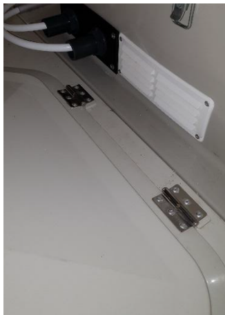
Example incorrectly sized weir on CWSTs
