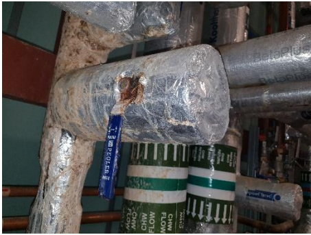
GENW11-068 Evidence of Leak
