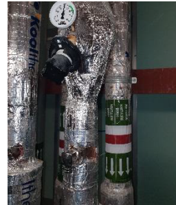
CC0-021 Deadlegs on Cold HF&R (Bottom)
