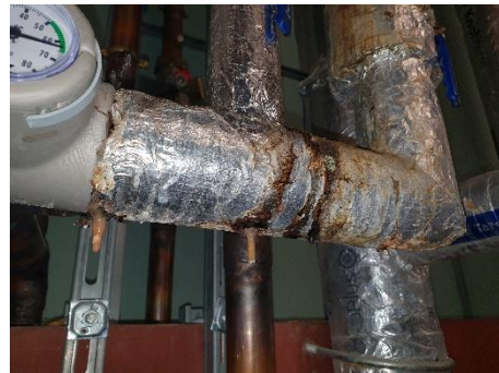
RENW-212 Evidence of Leak (1)
