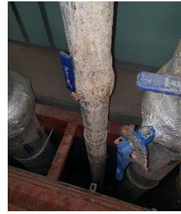
GENW11-068 Evidence of Leak (2)
