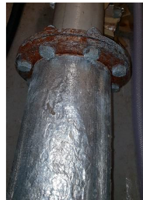
Example – non galvanised CWST steel supports
