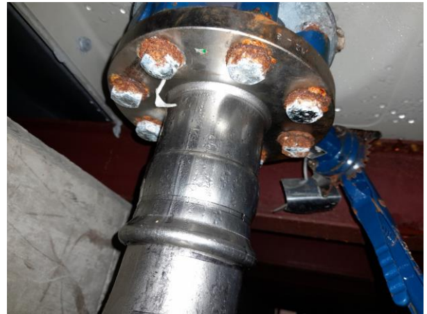
Example of CWSTs Fittings Condition
