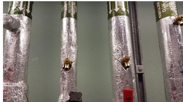
Riser Injection Points (Typical) (3)
