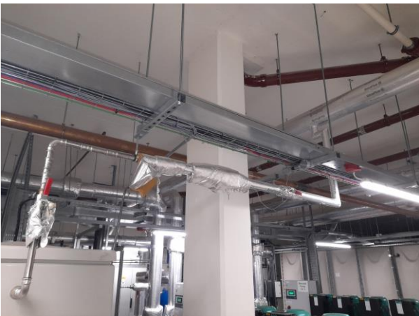
Position of DCV on Supply to Trade Water CWST 1 after Water Meter.
