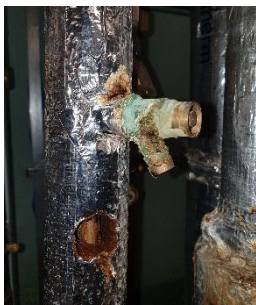
RCG-008 Unlabelled and Missing Insulation (2)
