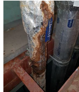
GENW11-068 Evidence of Leak (2)
