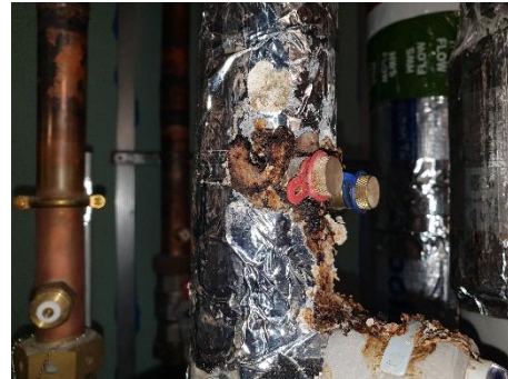
RENW-212 Evidence of Leak (1)
