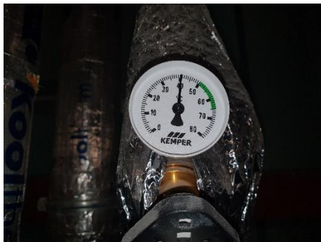
GENW6-068 Faulty Temp Gauge (2)
