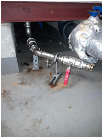
Example CWST Drain Points - Flushing Regime
