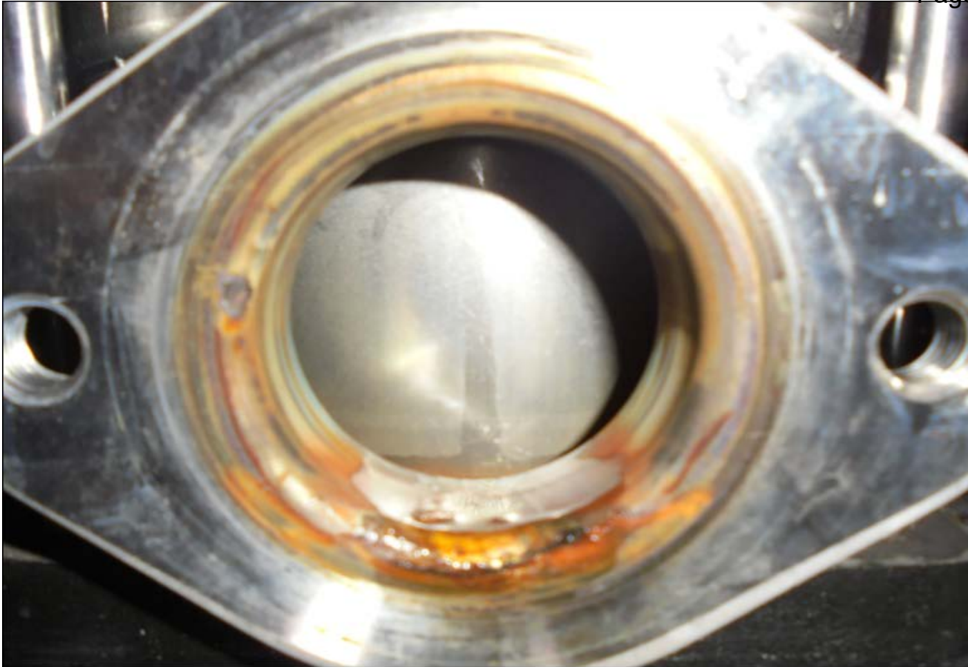
Fig 2 316, 1, 2 and 3 HWS Return Pump (internal)
