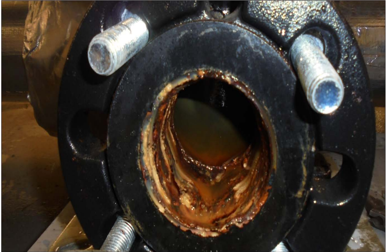
Fig 2 Booster Set 2 (Pump number 5) (Source NHS Scotland)
