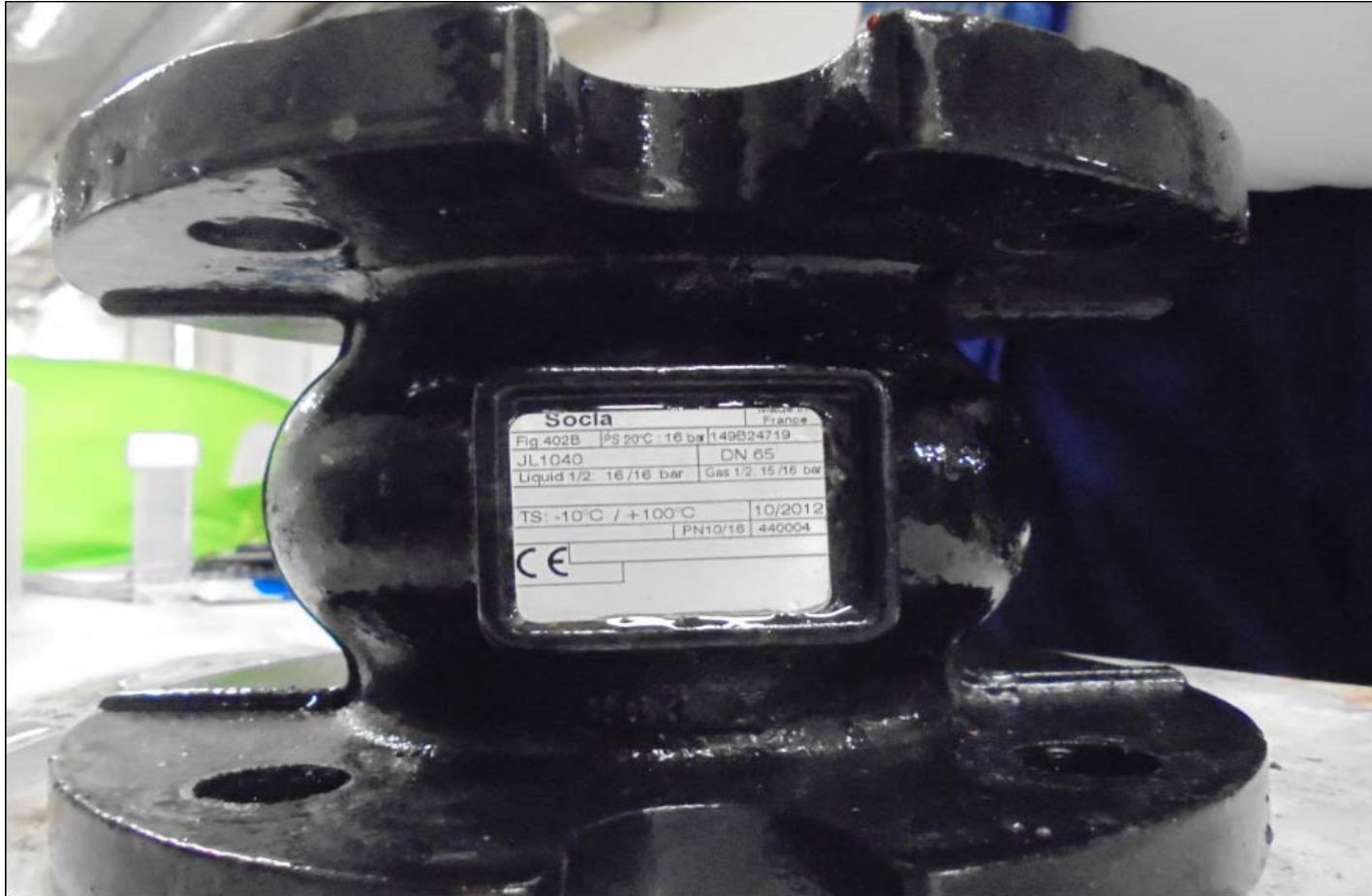
Fig 8 Booster Set 2 (Pump number 5 NRV Details)
