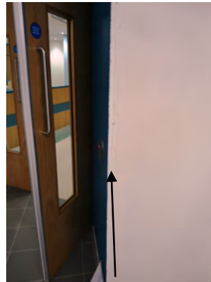
Damaged corner bead
