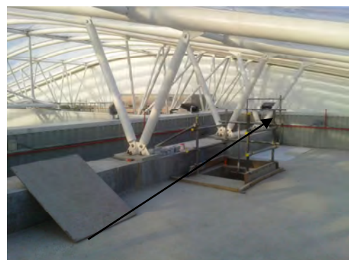
Temporary scaffolding providing perimeter protection.
