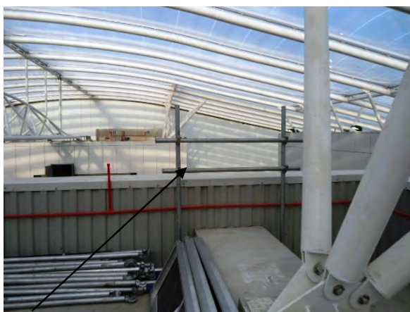
Temporary scaffolding providing perimeter protection.
