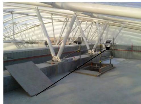
Temporary scaffolding providing perimeter protection.
