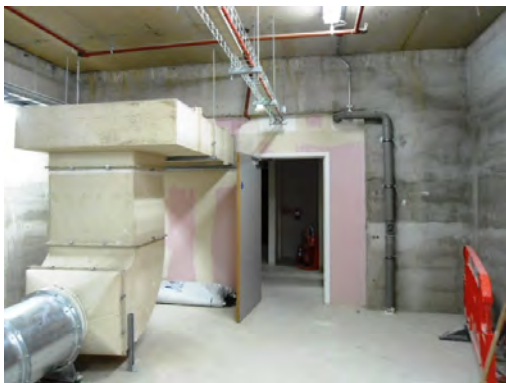
Level 12 Core A incomplete work.
