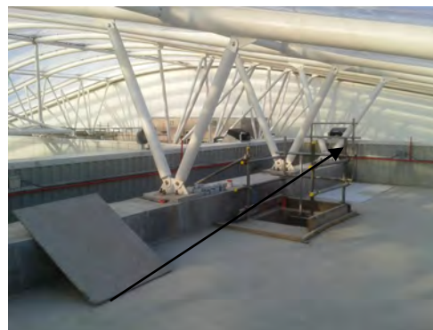
Temporary scaffolding providing perimeter protection.
