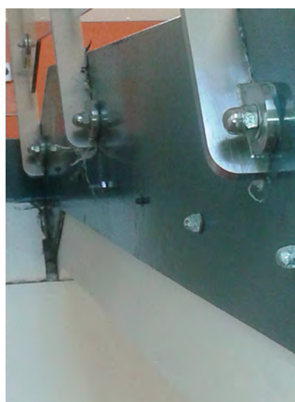
Nuts still to be cropped and fitted to steel stringer.
