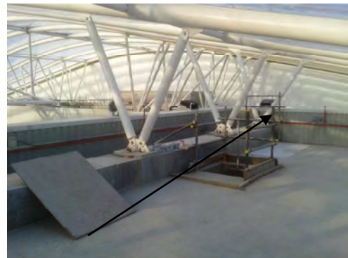
Temporary scaffolding providing perimeter protection.
