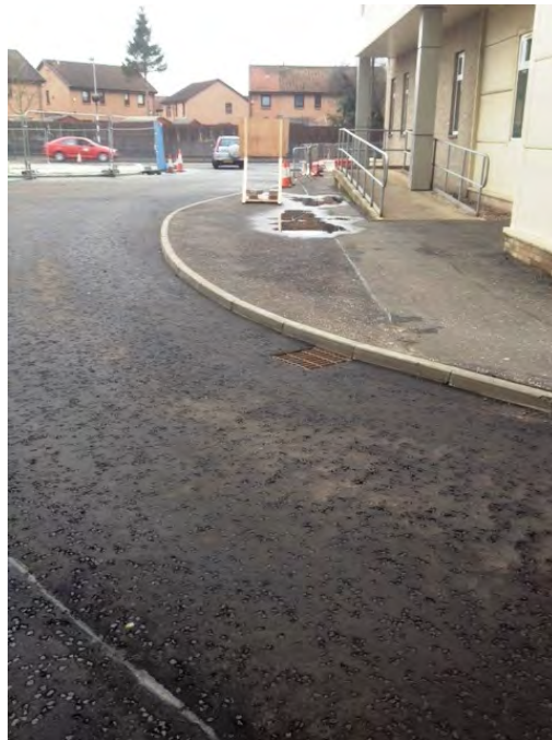
Footpath to the east side of the maternity unit.
