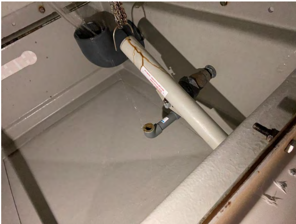
Corrosion at inlet valve and surrounding stainless steel components image 016
