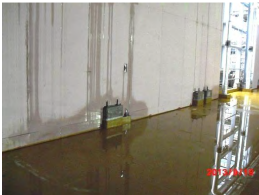
Water damaged boards.
