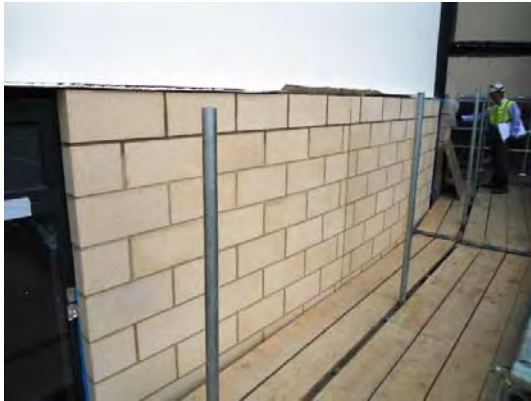
Blockwork at the Children's Hospital.
