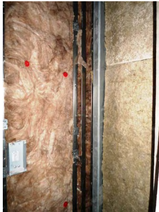
Junction of partition with external wall
