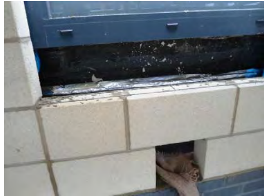
Reinforcing at window.
