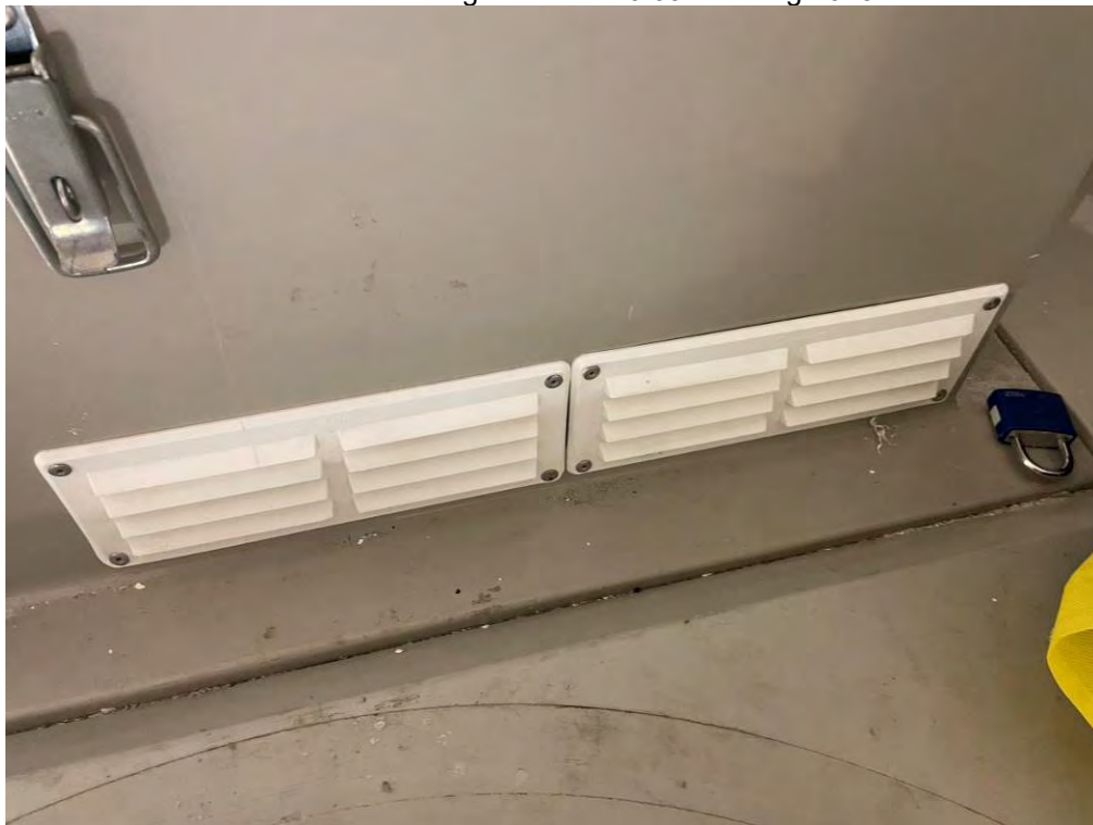
Air intake vent with screened mesh greater than 0.65mm image 019
