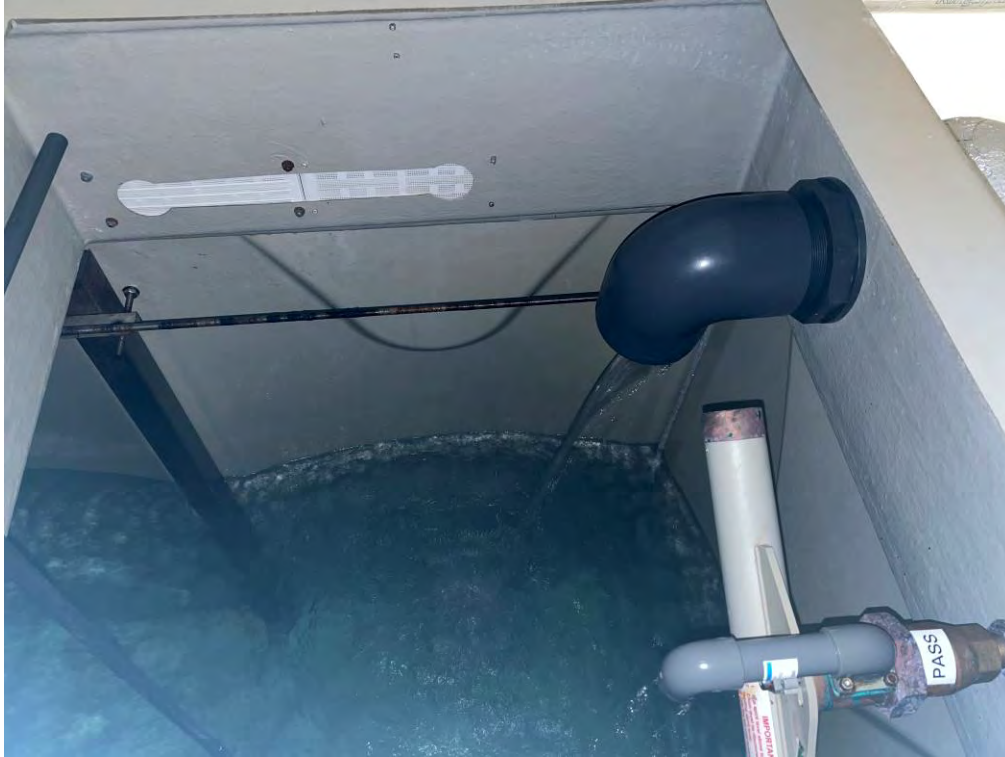
Corrosion at inlet valve and surrounding stainless steel components image 016
