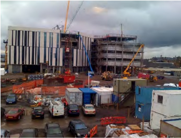
8. Cladding at Front Elevation.
