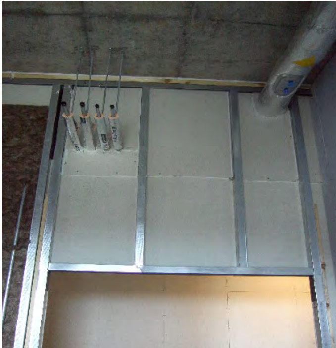
6. Example of Shaftwall installation.
