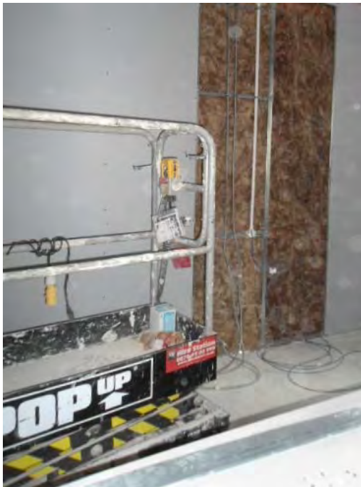
Insulation in partition.
