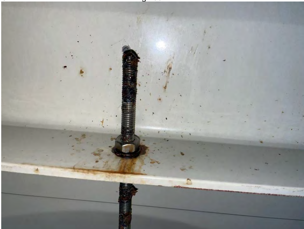
Corrosion of internal stainless steel image 004
