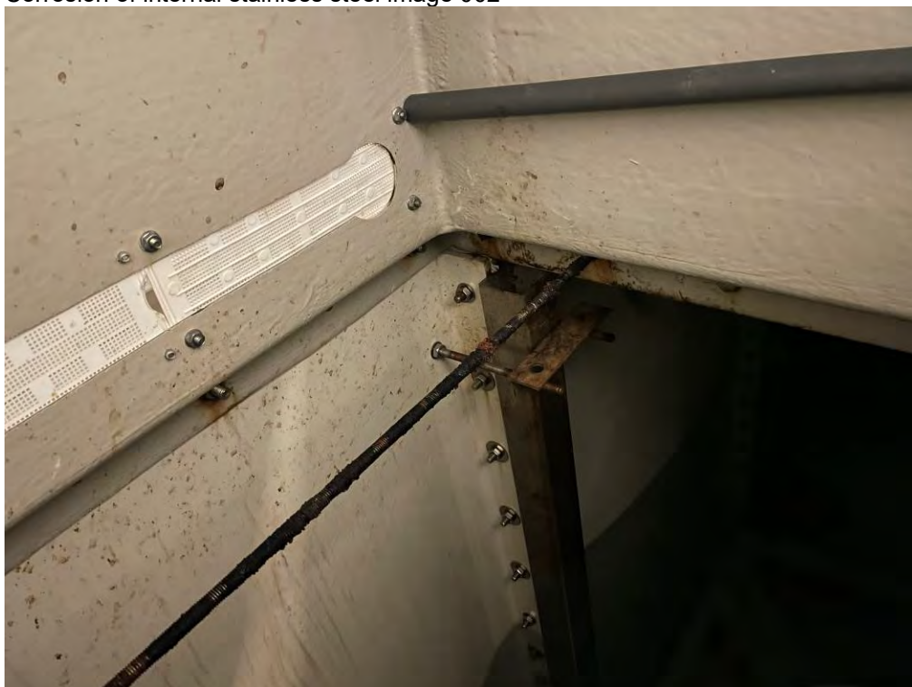
Corrosion of internal stainless steel image 002
