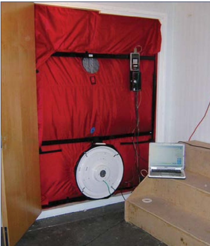
Figure 1: Flow pressurisation equipment during air permeability testing of an isolation suite
