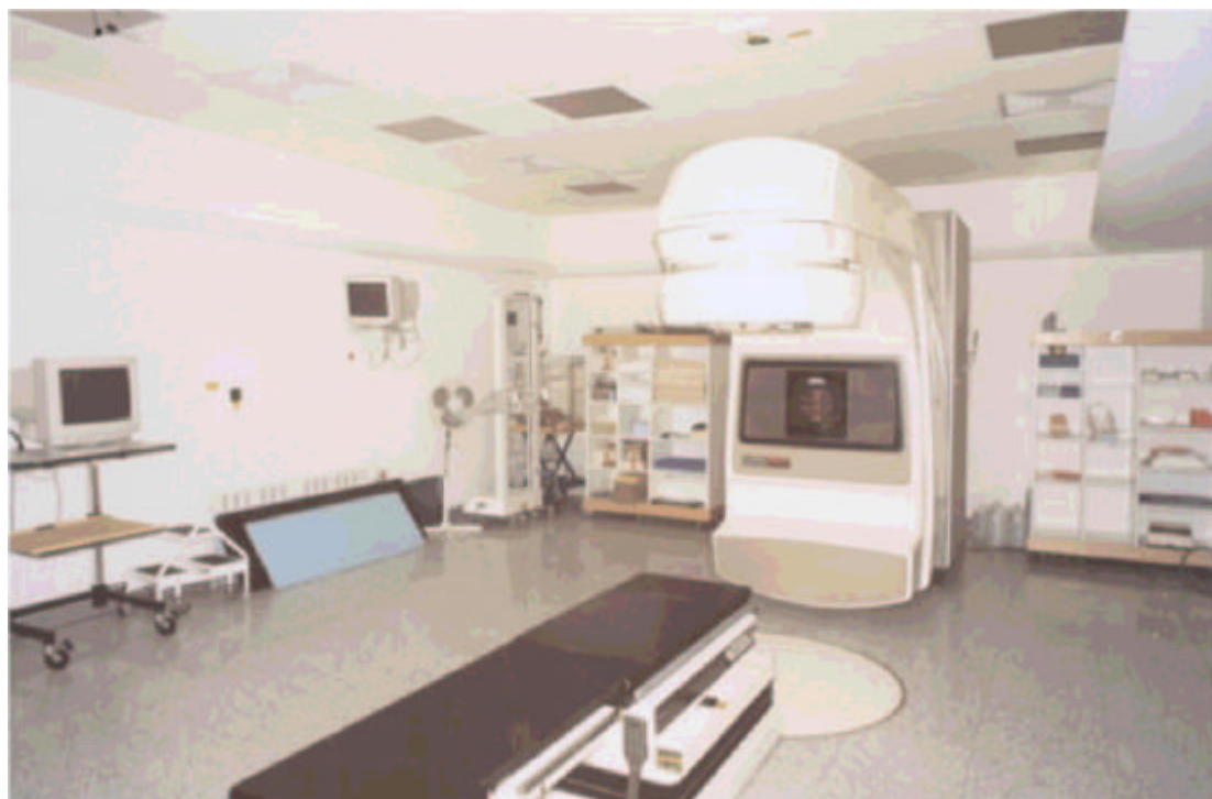
Linear accelerator treatment room showing treatment gantry with enclosed machine cabinet
