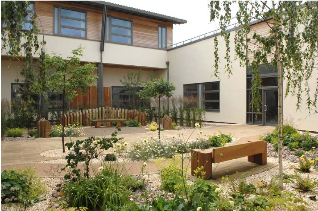
Figure 6: Courtyard, Queen's Centre for Oncology & Haematology, Hull (Reproduced with the permission of HLM Architects – photographer Ian Bruce)
