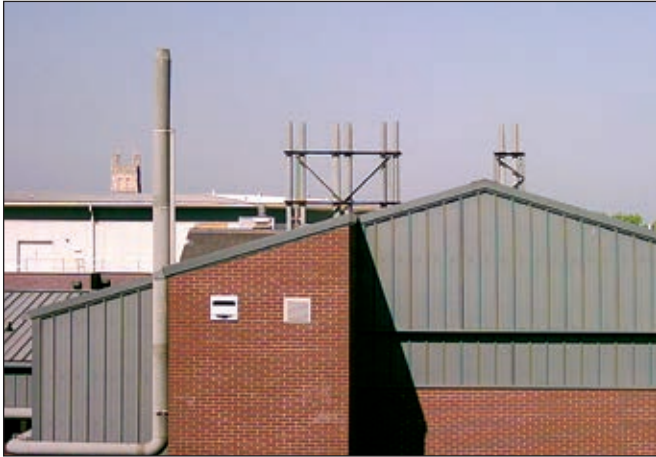
Typical LEV discharge stacks
