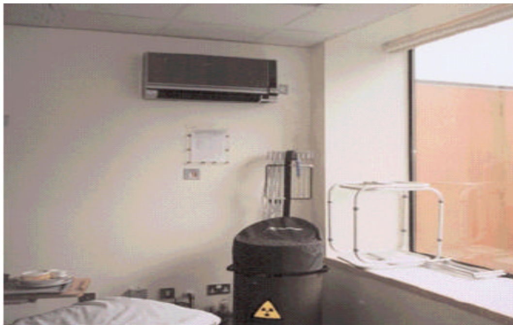
Single bed LDR/MDR treatment room showing window in external shielding wall. Shielding continuity is maintained by use of a free-standing concrete shielding wall enclosing a controlled area that can be landscaped for the benefit of the patient.
