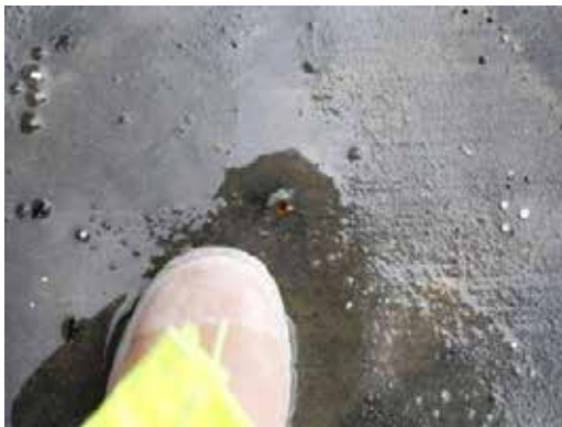
Damaged Membrane
