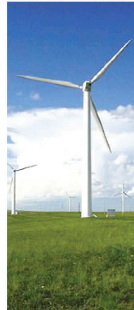
An 80m Turbine
