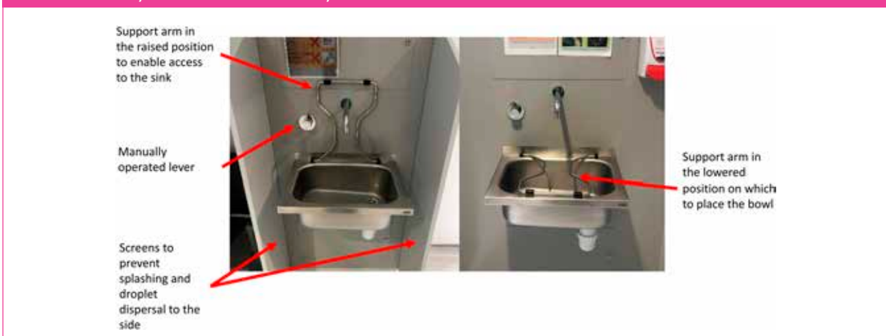
Figure 3. Use of a support arm. Note: This innovative design was developed at the Norfolk and Norwich University Hospital NHS foundation Trust by Sarah Morter and Marc Lillystone
