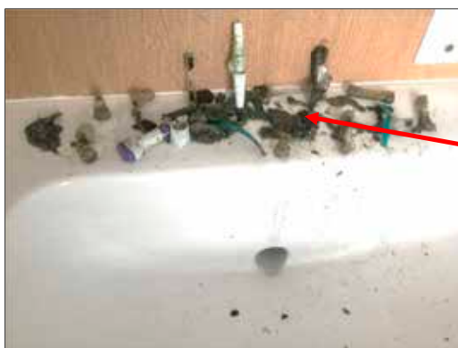
Figure 3. Example of debris removed from the u bend.
