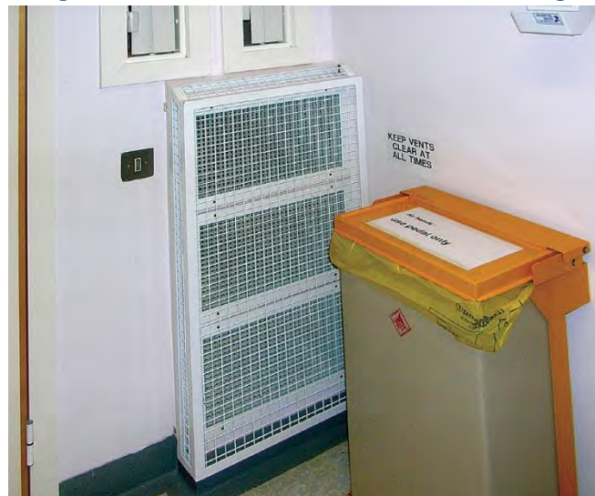
Figure 8 Pressure stabiliser with stand-off cage
