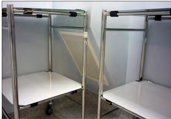
Figure A27 Low level extract recommended installation
