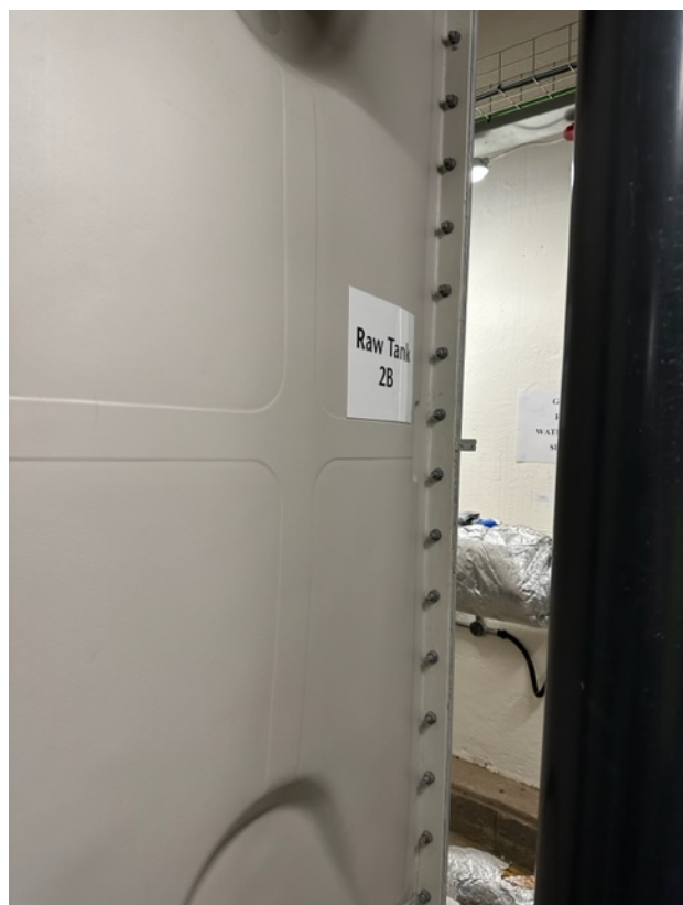
Figure 9. Raw water storage tank 2B.
