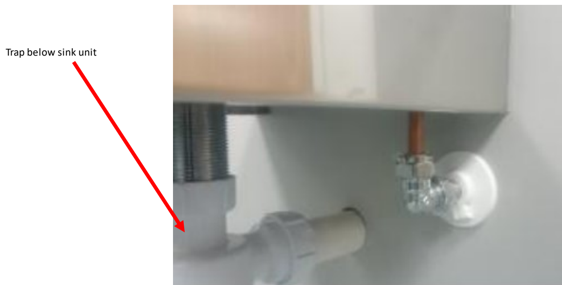
Figure 23. Position of trap below a sink unit.
