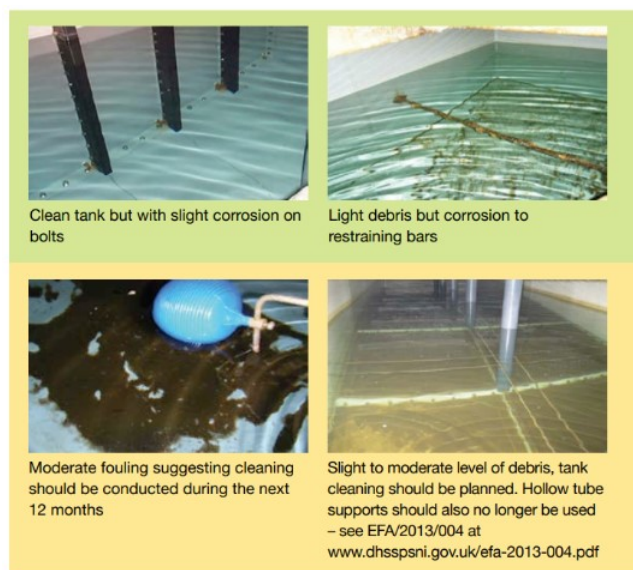
Figure 35. Sediment deposition on the floor of a cold water storage tank as identified in HSG 274.
