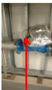
EPDM flexible hose to dishwashers
