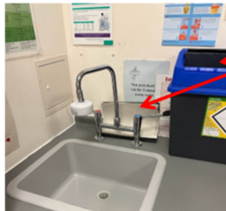
Figure 58. Corner sink unit will be underused and items on countertop will be splashed leading to surfaces contamination and biofilm under the container
