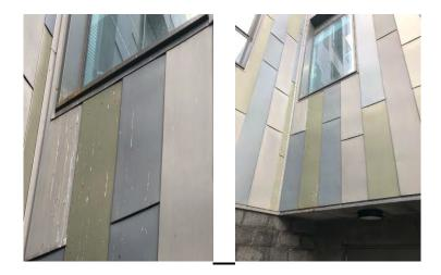
Pigeons are roosting on 8 ledges we recommend removal of all pigeon fouling, sanitisation of area with a biocide then installation of bird repellent spike to roosting site works would be carried out from specialised access equipment.
