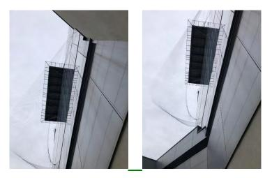
Pigeons are gaining access due to damaged netting. GP Environmental recommend a Specialised Environmental Deep Clean of all pigeon fouling followed by the sanitisation of area with a biocide then a repair of bird repellent netting to prevent any further contamination.
