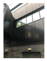
Pigeons are roosting on 2 exposed ledges we recommend removal of all pigeon fouling, sanitisation of area with a biocide then installation of bird repellent spike to roosting site works would be carried out from specialised access equipment.
