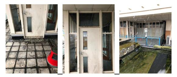
Pigeons are roosting above doorways and on all ledges we recommend removal of all pigeon fouling, sanitisation of area with a biocide then installation of bird repellent nets at the rear of Maternity Building.
