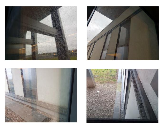
Pigeons are roosting on the external high level ledges in this area. GP Environmental recommend a Specialised Environmental Deep Clean of all pigeon fouling followed by the sanitisation of area with a biocide then installation of bird repellent mesh to roosting site to prevent any further contamination.
