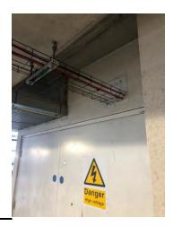
Pigeons are roosting on cables and ledges above we recommend removal of all pigeon fouling, sanitisation of area with a biocide then installation of bird repellent spike to roosting site.
