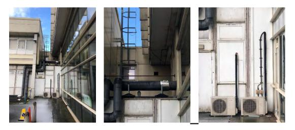
Pigeons are roosting and nesting within the void area we recommend removal of all pigeon fouling, sanitisation of area with a biocide then installation of bird repellent netting to prevent further ingress by pigeons.
