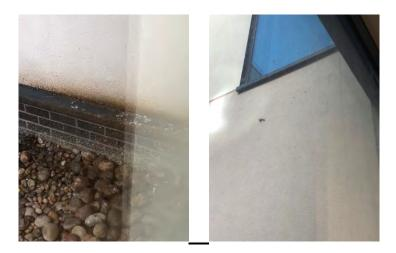
Pigeons are roosting on ledge above we recommend removal of all pigeon fouling, sanitisation of area with a biocide then installation of bird repellent spike to roosting site
