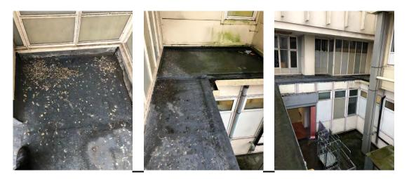
Pigeons are roosting and nesting in void corner we recommend removal of all pigeon fouling, sanitisation of area with a biocide then installation of bird repellent nets to prevent further ingress from pigeons.
