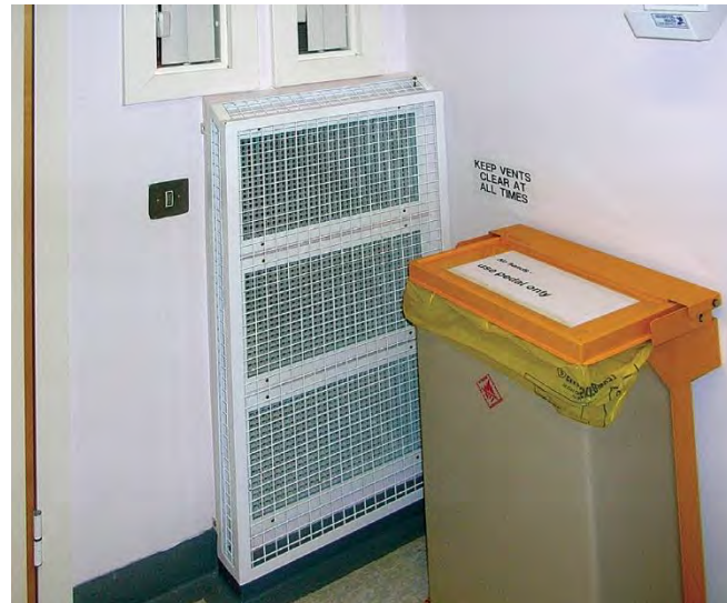
Figure 8 Pressure stabiliser with stand-off cage
