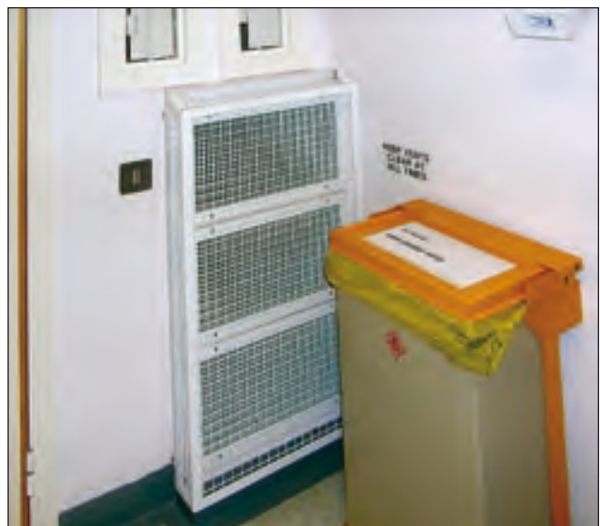
Pressure stabiliser with stand-off cage
