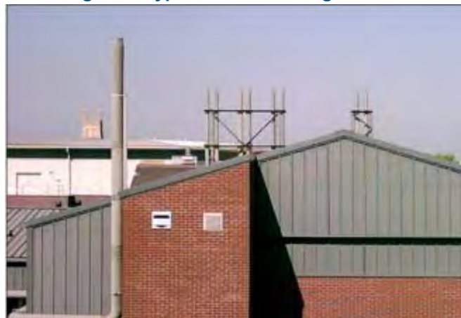
Figure 9 Typical LEV discharge stacks
