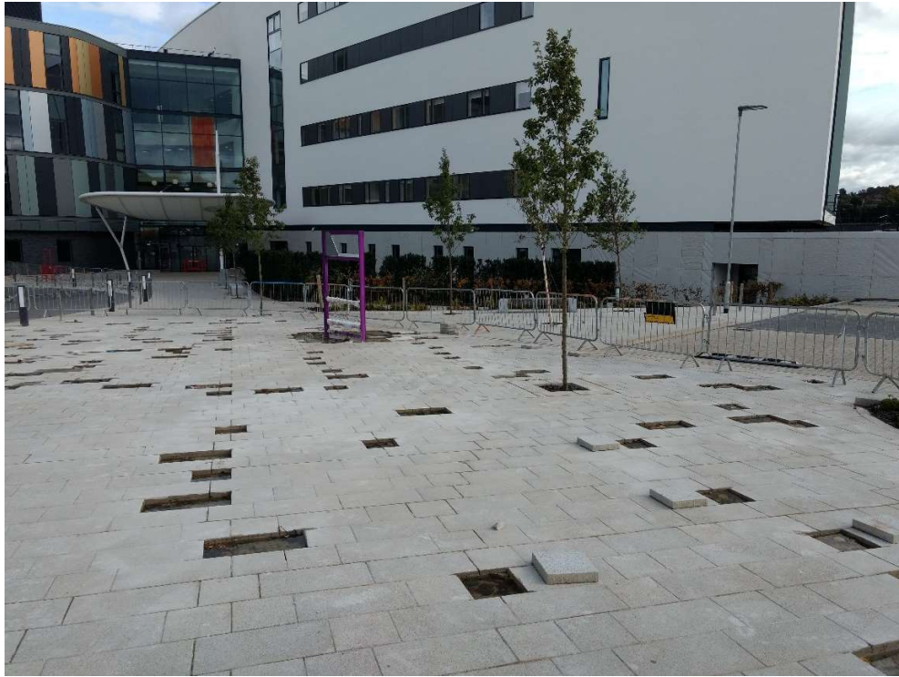
4 – Extent of replacement slabs to main entrance
