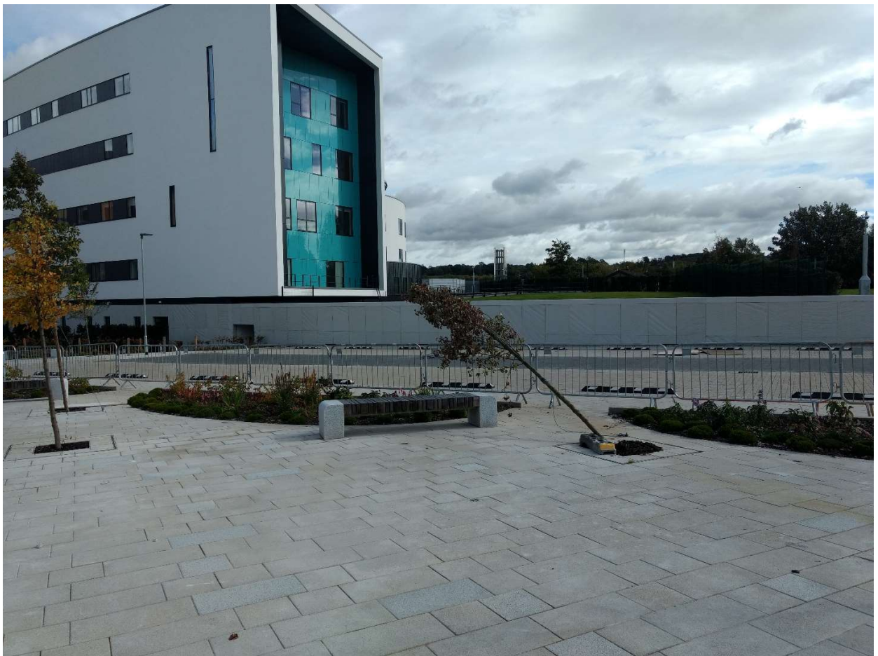
6 – Numerous trees have sustained wind damage
