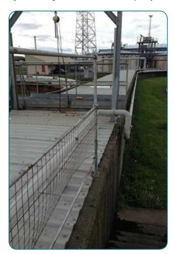
Figure 5: Chemical scrubber for air extracted from inlet works and primary tanks
