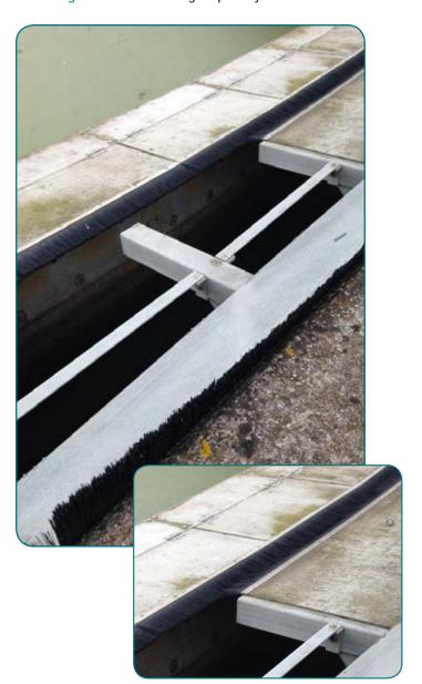
Figure 4: Covering on channel from inlet works to primary tanks
