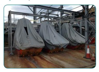
Figure 3: Brush covering on primary tank weirs
