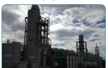
Figure 6: Activated carbon scrubber for air extracted from thermal hydrolysis sludge plant
