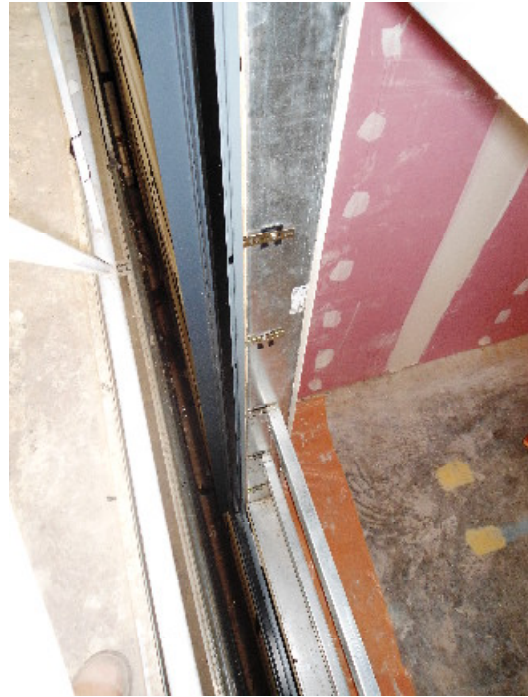
Internal fixing to windows
