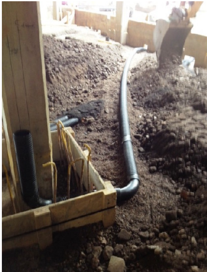
Photo 4 – Storm water drainage run in Zone D
