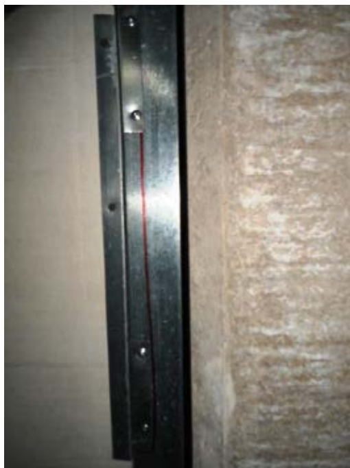
Vertical stud not tight to the column.
