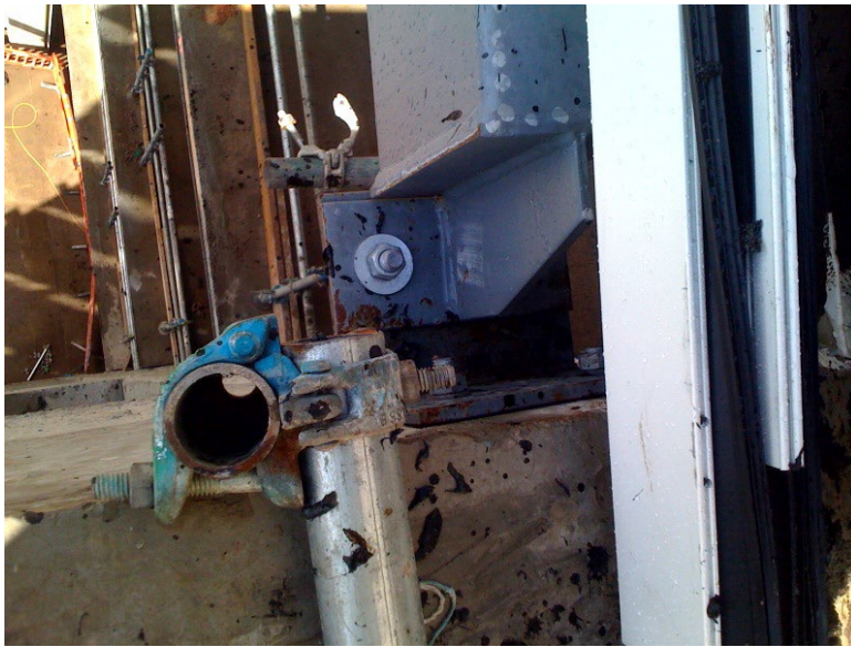
14. Solution to overlap of bolt head May 2011.
