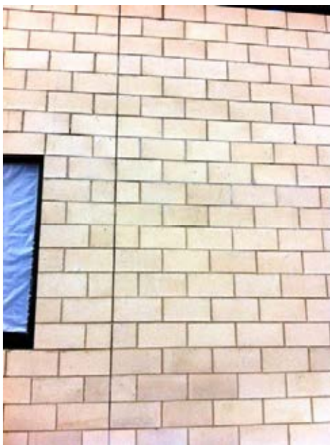
Inconsistent pointing both colour and quality.
