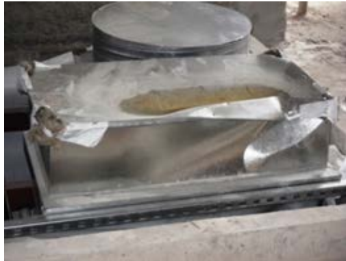
Damaged duct Level 3 Plant Zone D
