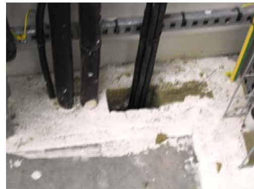
Gap in the fire bat in room GEN21-054
