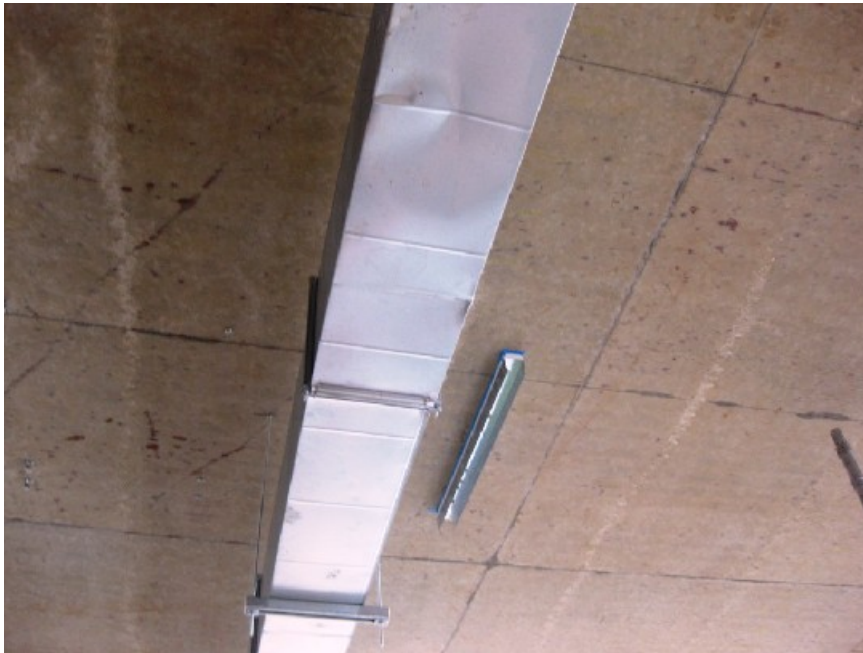
Photo No 1. Damaged trunking on Level 1.
