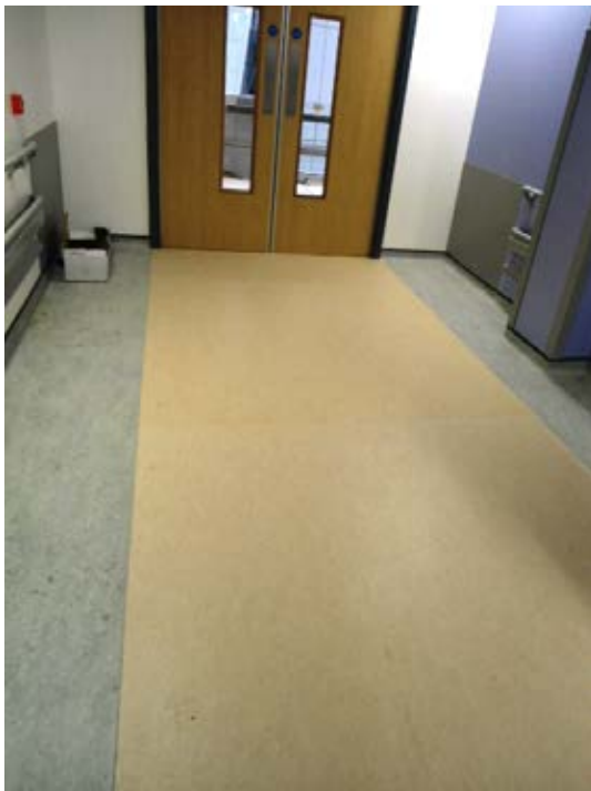
Shading on newly fitted vinyl.
