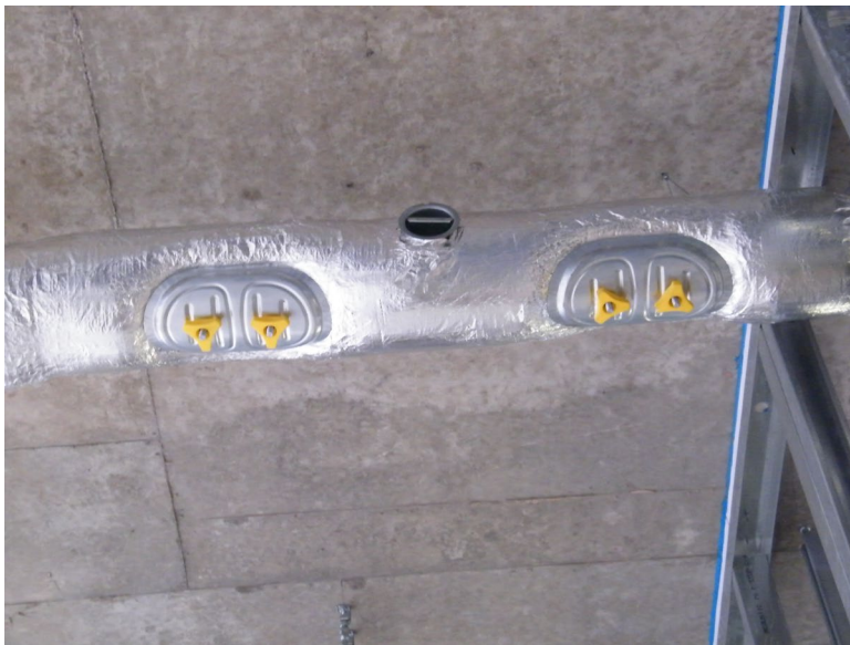
7. Inspection doors fitted over insulation May 2011.
