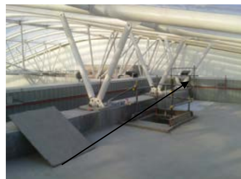
Temporary scaffolding providing perimeter protection.
