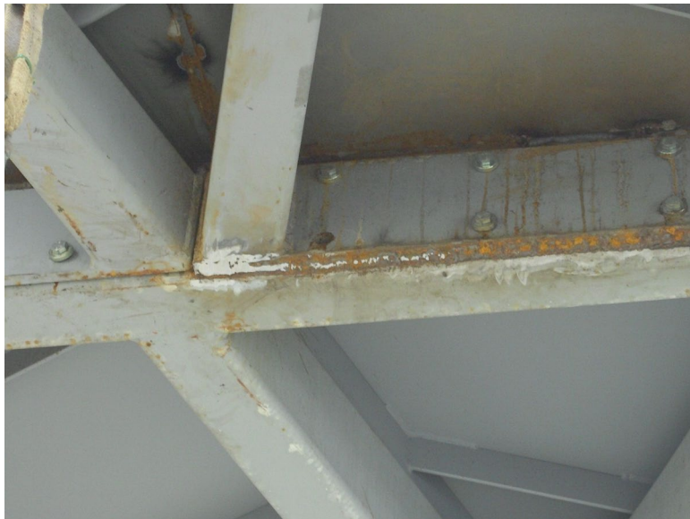
3. Missing bolt at Pod stair April 2011.
