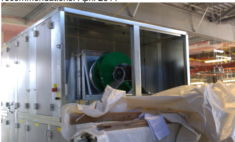
9. Unprotected AHU. April 2011
