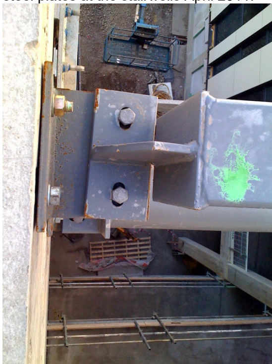
11. Tight bolt head to hole overlap April 2011.
