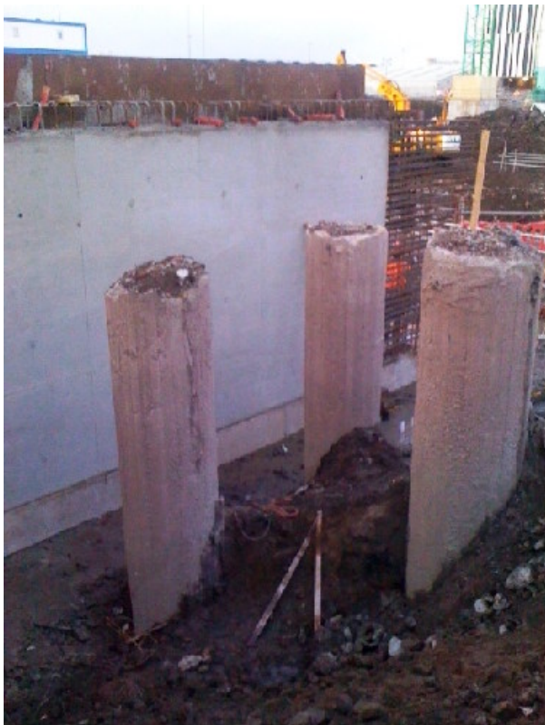
Piles out of alignment
