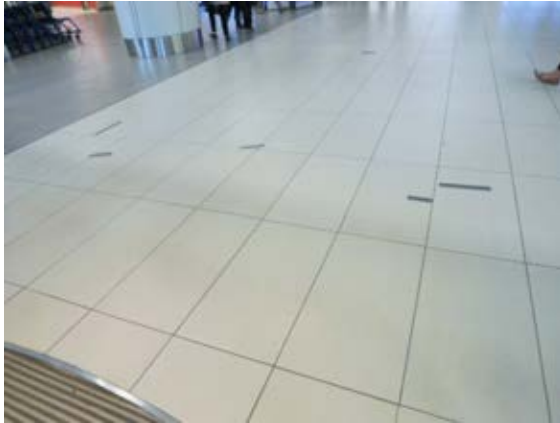
Damaged tiles at main entrance.
