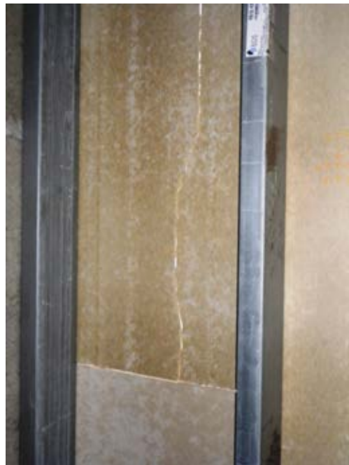
Crack in board.
