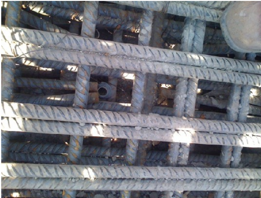
Photo No 7. Congested reinforcing.
