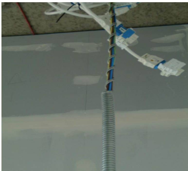
10. Damaged flexible conduit May 2011.
