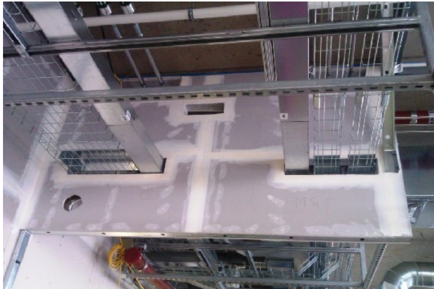
Photo 5. Partition Formed around Services.
