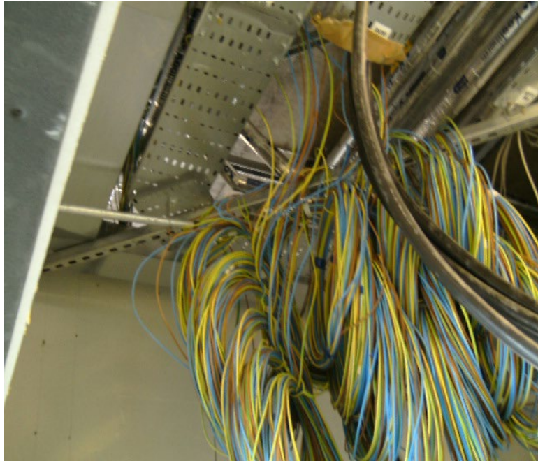
12. Cable protection required May 2011.
