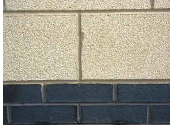
Damaged edge of blockwork at perpend.
