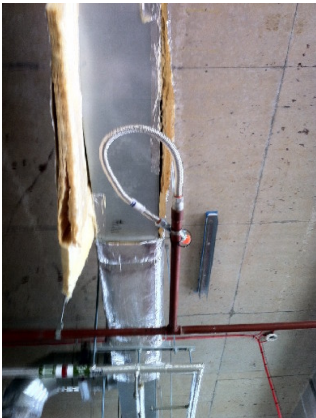
Photo No 2. Section of damaged trunking show above replaced.
