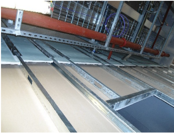
Photo 5 – Insulation not fitted to shaftwall.
