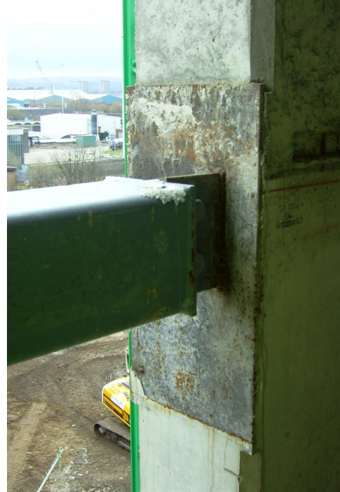
2. Rust on steel plate.
