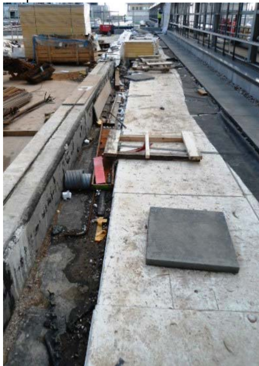
Debris and materials on the roof which could damage the protective membrane.
