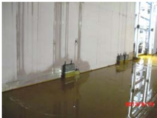
Water damaged boards.
