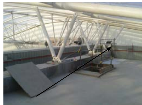
Temporary scaffolding providing perimeter protection.
