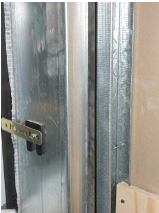
No insulation behind partition.
