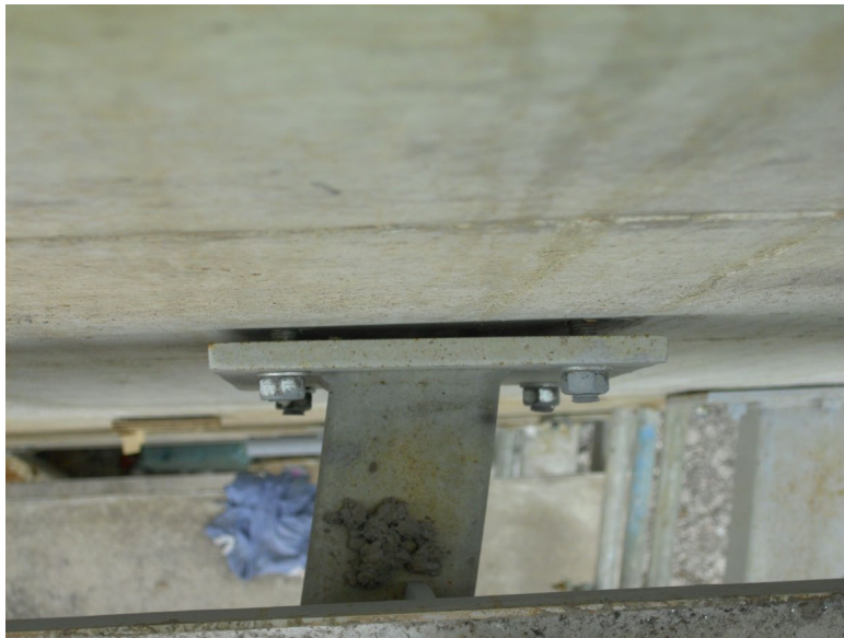
4. Gap between wall and plate at Pod Stair April 2011.
