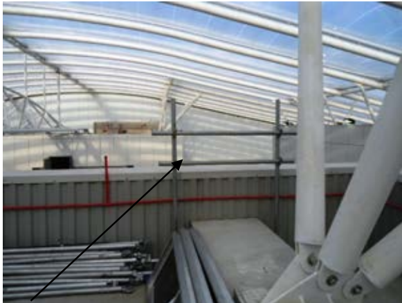
Temporary scaffolding providing perimeter protection.
