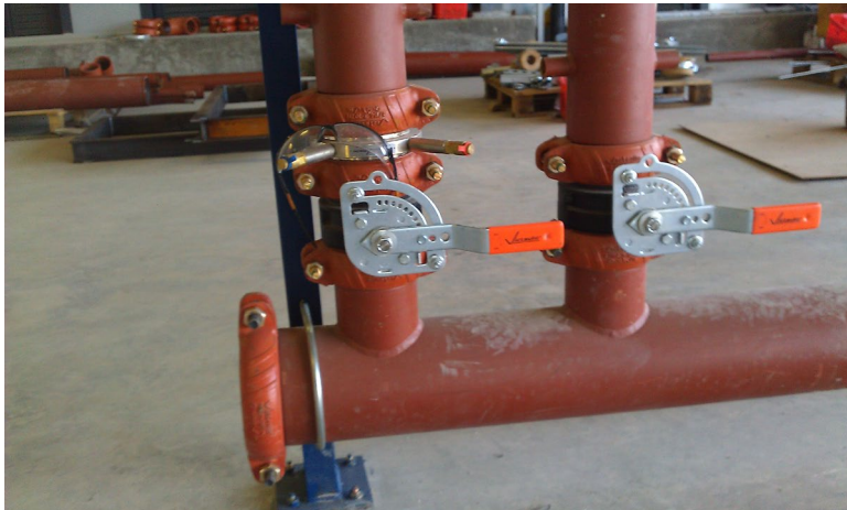
8. Commissioning Set not installed as manufactures recommendations. April 2011.
