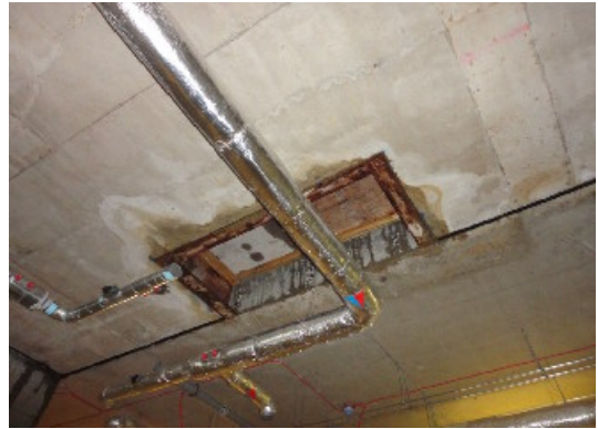
Water ingress as a result of rain penetration through soffit.
