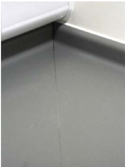
Poorly fitted joint to worktop recorded on Brookfield's IDMS
