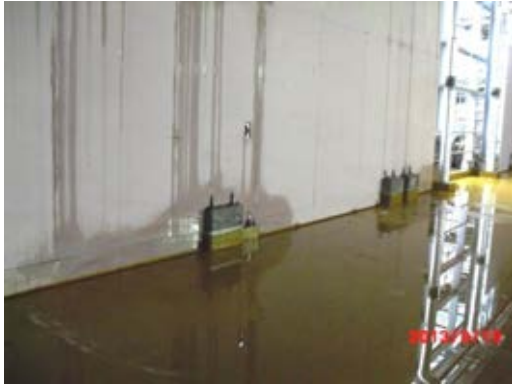
Water damaged boards.
