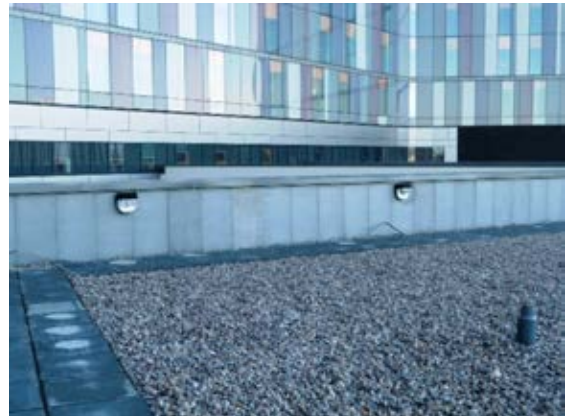
Roof R5-005: Roof lighting lightning still to be wired and conductor tape still to be fitted.
