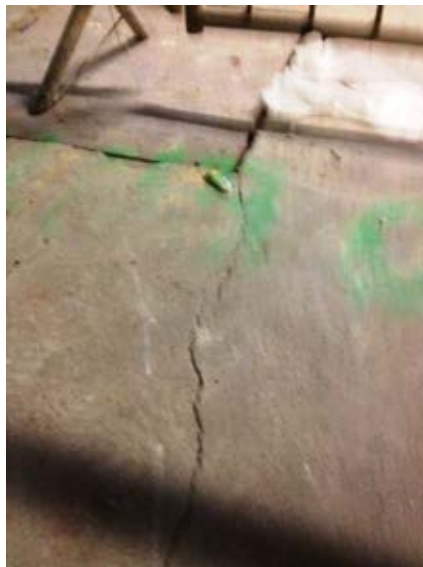
Cracks in Level 0 floor
