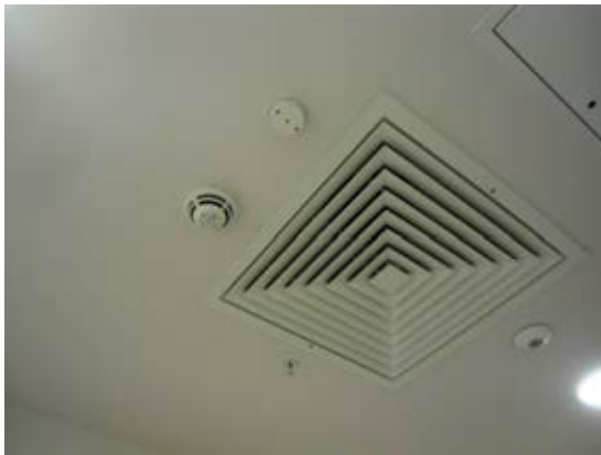
Smoke detector too close to air supply vent.
