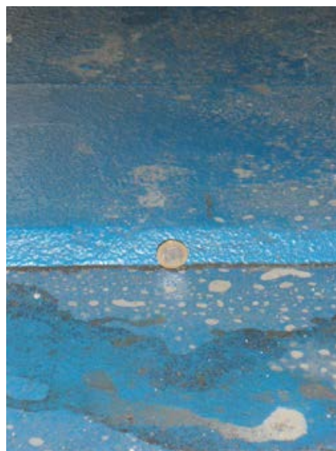
Level 3: Channel exceeds 30mm deep.
