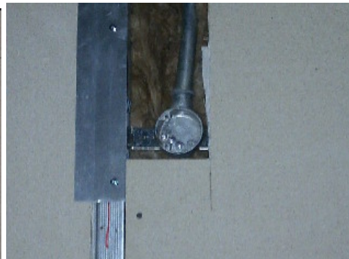
Services moved and stud strengthened.
