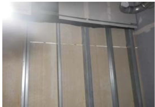
Excessive joint in boards.
