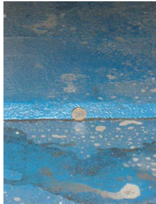
Level 3: Channel exceeds 30mm deep.
