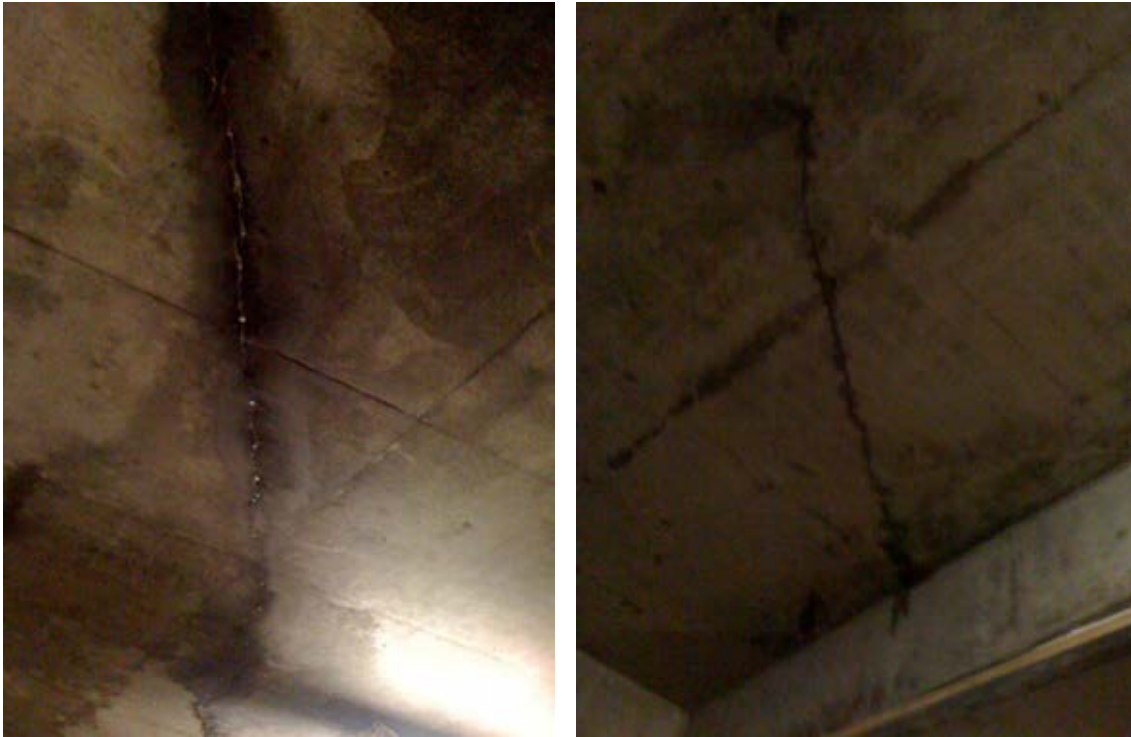
3. Crack in Water Tank Area: 14 th December 2010.
