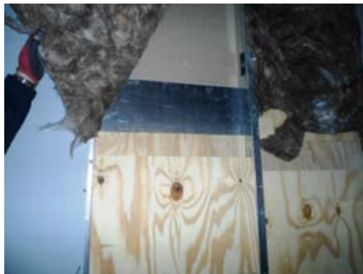
Insulation missing behind pattresses.
