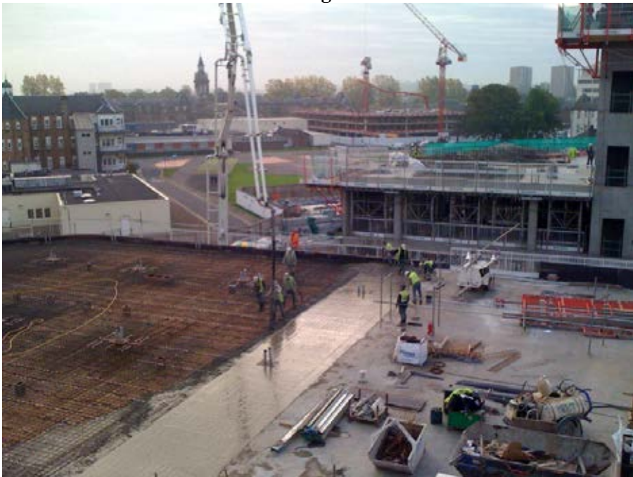
4. Mortuary 1 st floor slab pour: 14 th October 2010
