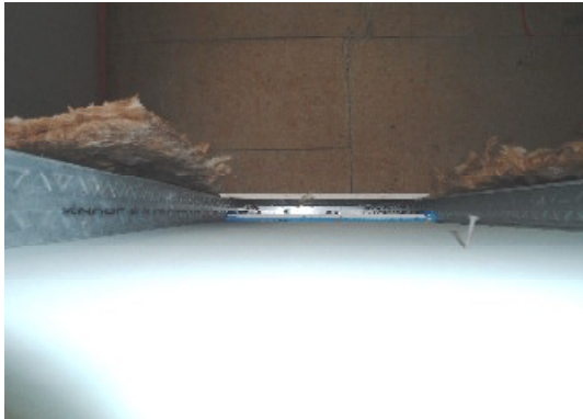
Room CCU-068. Insulation missing at high level
