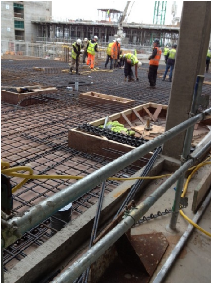
Photo 5 – Steel fixing to slab being cast.
