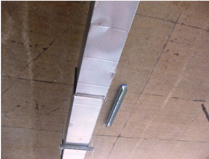
Photo No 1. Damaged trunking on Level 1.
