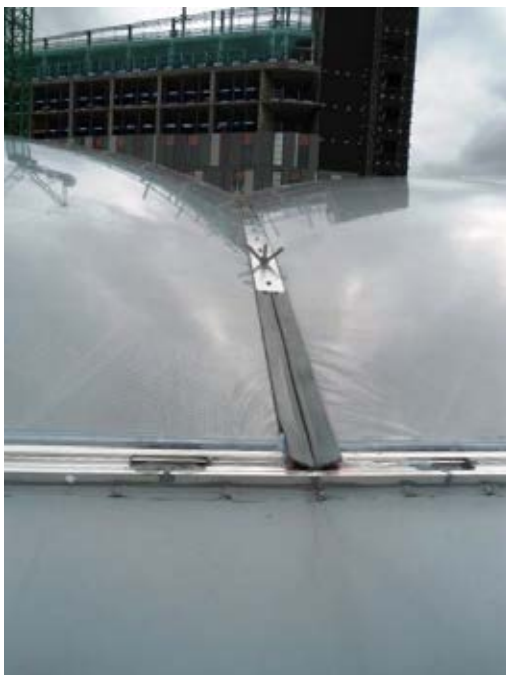
Joint section at Barrel Vaulted Roof.
