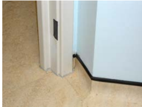
Weld not completed.
