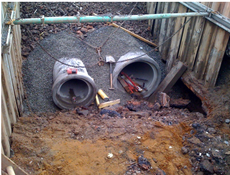
15. Gully positions adjacent to the outside edge wall. Falls readily to be feed to these positions may 2011.
