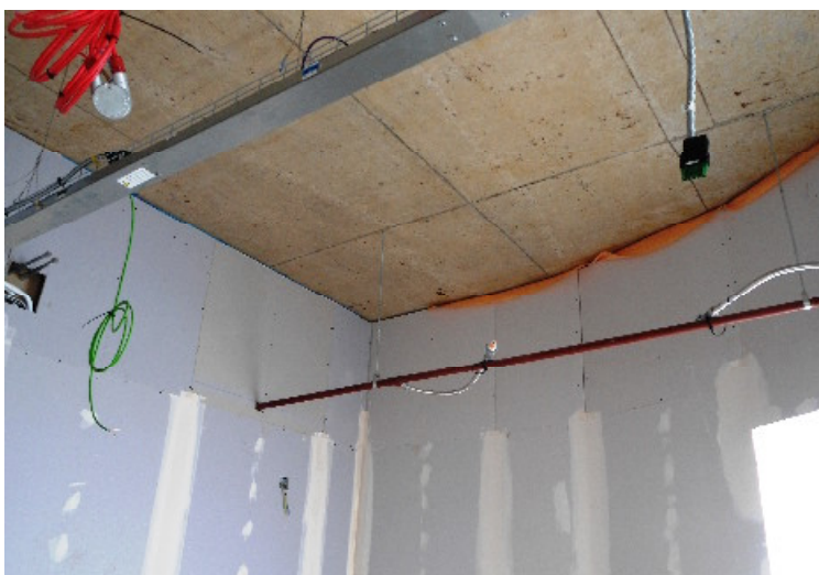
Photo 6 – horizontal joints not in accordance with NBS specification
