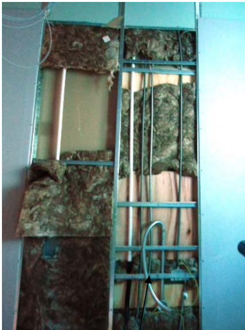
Insulation missing behind pattress
