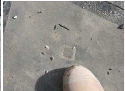
Indent in protective membrane.
