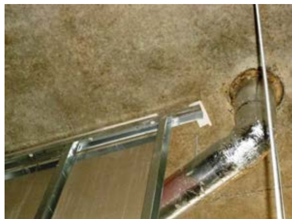
Sealant missing at headtracks.
