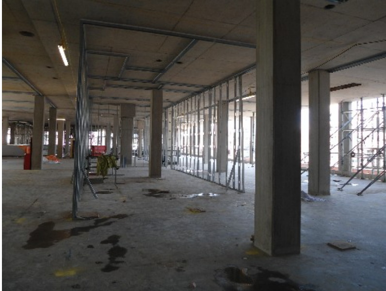
Photo 1 – Partitions being erected on Level 1 area 529 Zone H.
