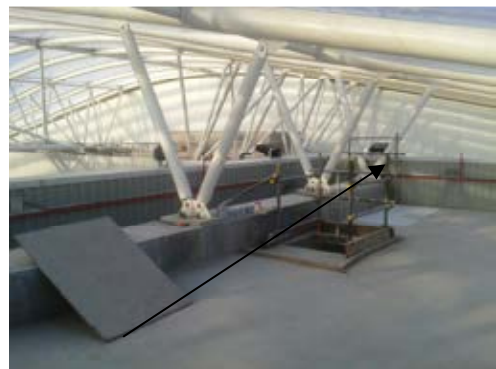
Temporary scaffolding providing perimeter protection.
