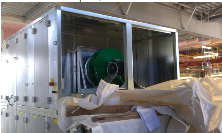
9. Unprotected AHU. April 2011.
