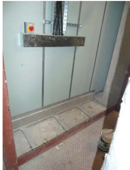
Gap between the metal deck and the wall with the floor comprising fire bats.
