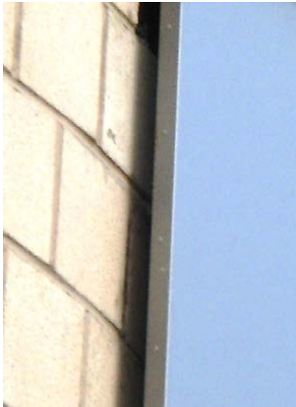
Gap between cladding and blockwork interface.
