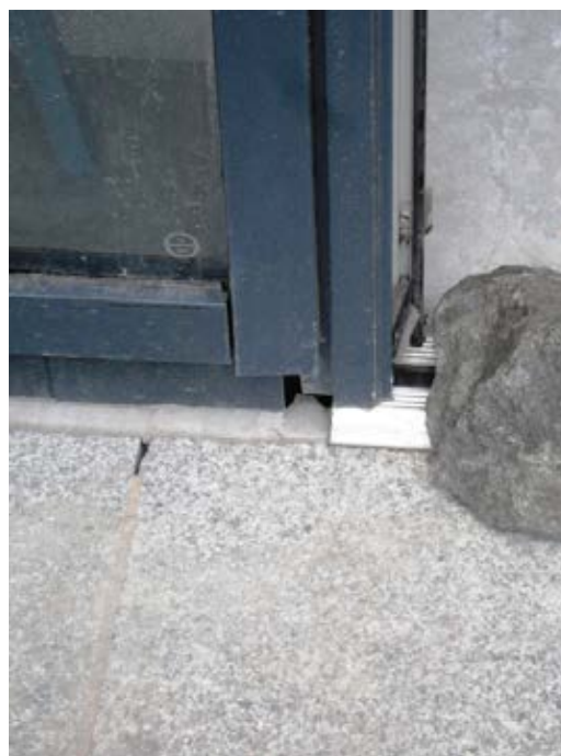
Excessive gap at the bottom of the door frame.
