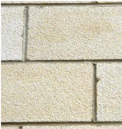
Damaged blockwork and overspill of mortar pointing at edge of blockwork.
