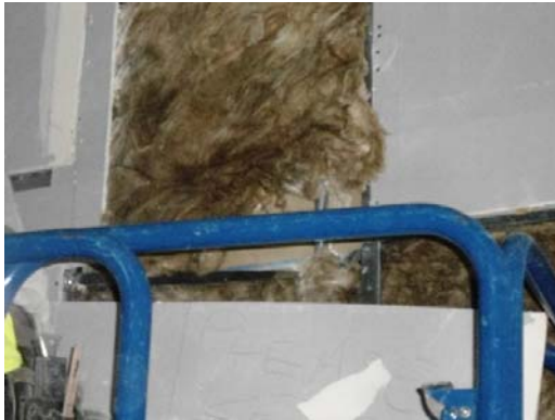
Insulation disturbed behind the boarding.
