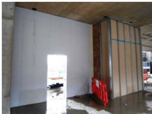
Water damaged boards.
