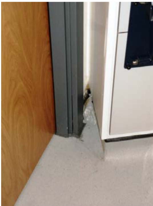
Poor vinyl detail at recess.
