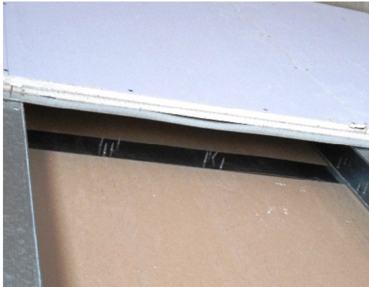
Photo 1 – Upper section of partition without insulation
