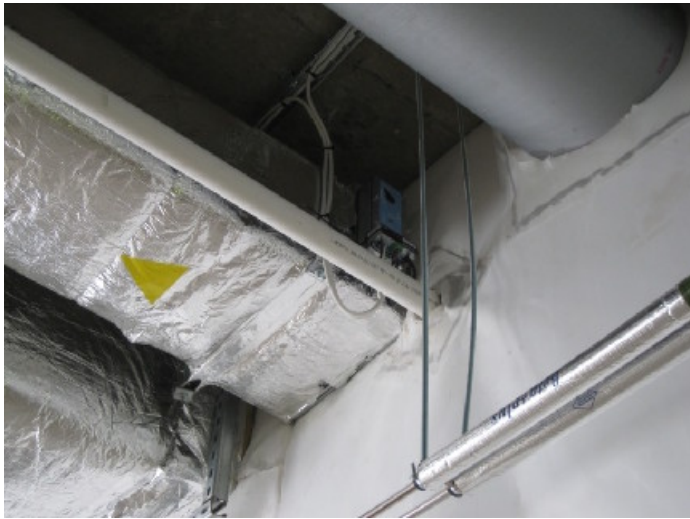
Photo 3 – Ductwork with Motorised Damper Installed
