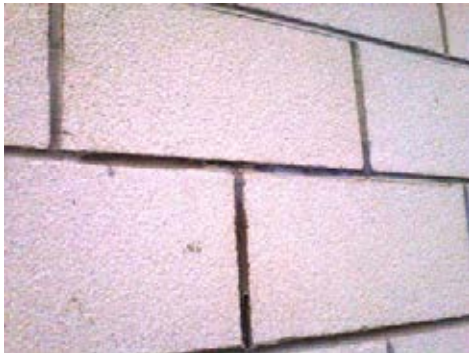
Inconsistent pointing both colour and quality.
