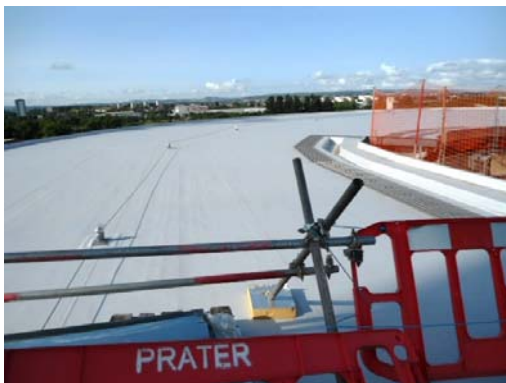
Finished Area of Sarna Roof
