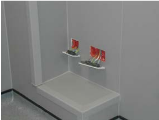
Fire putty present behind cover plate.
