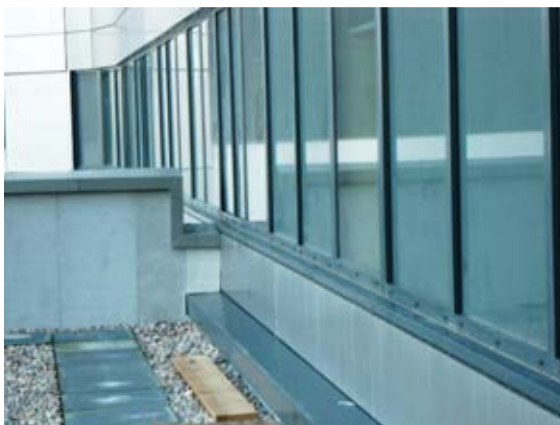
Lightning conductor tape not fitted.
