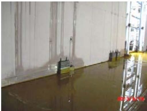
Water damaged boards.
