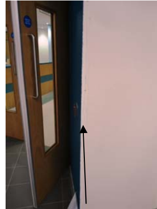
Damaged corner bead
