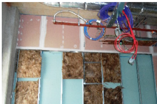
Room CCU-068. Partition with insulation missing at high level
