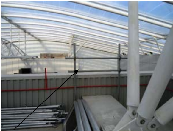
Temporary scaffolding providing perimeter protection.
