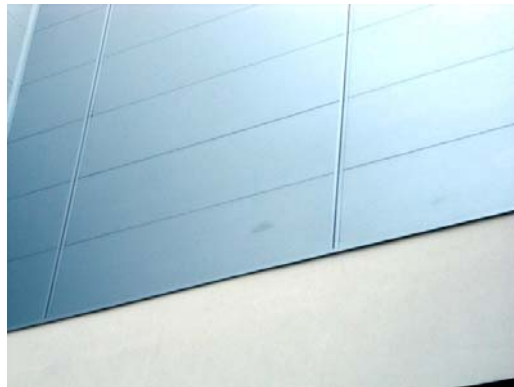
Unsuccessful repairs to cladding in Courtyard 3.
