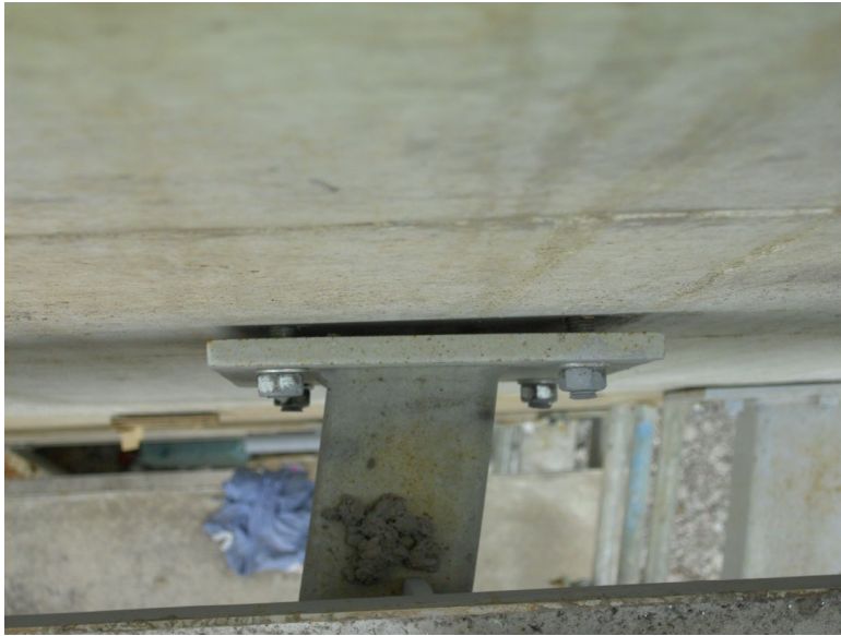
4. Gap between wall and plate at Pod Stair.
