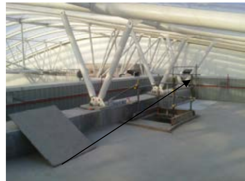
Temporary scaffolding providing perimeter protection.
