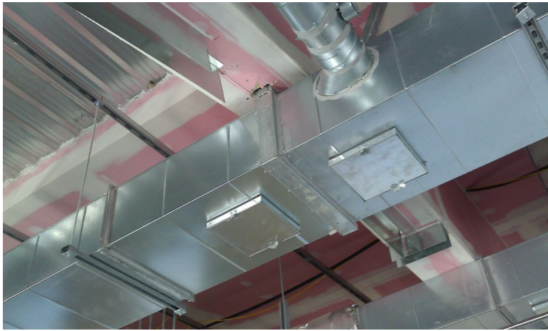
7. Fire damper in beam. April 2011.
