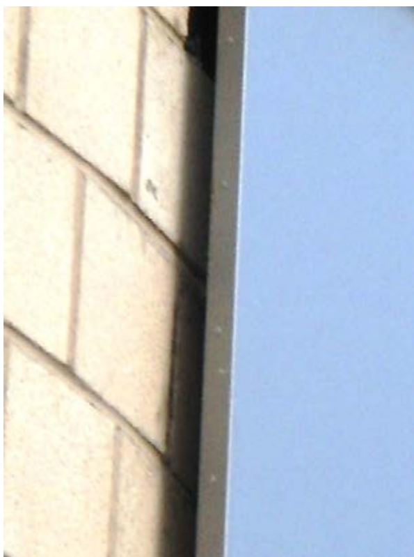
Gap between cladding and blockwork interface.
