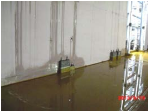
Water damaged boards.
