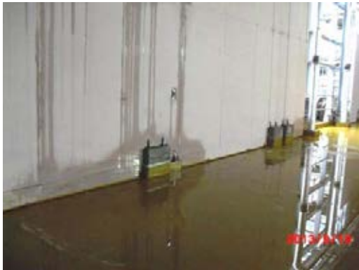
Water damaged boards.
