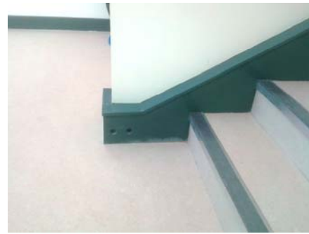
Holes to be filled in metal stringer.
