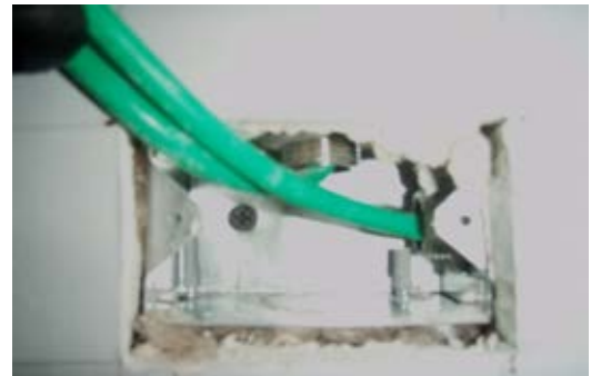
Rubber sleeves over screws.
