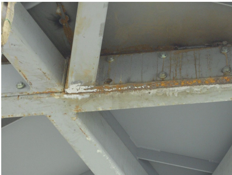
3. Missing bolt at Pod stair.
