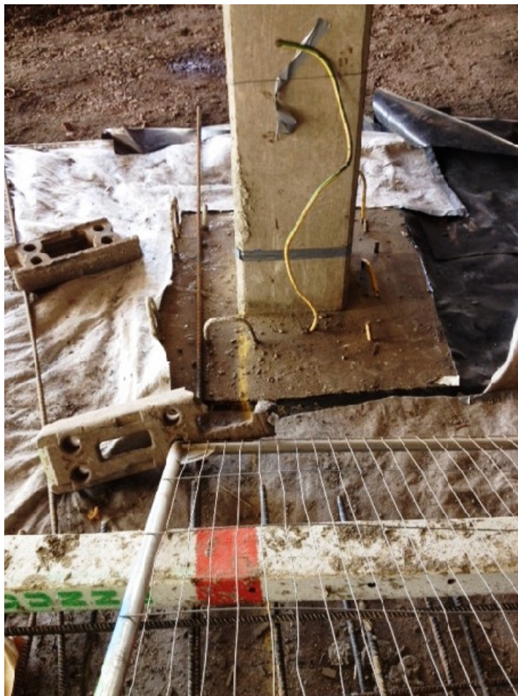
Photo 4 – Link reinforcement from pile caps Zone D.
