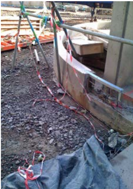
2 & 3. DPC Around Pod Floor Slab: 19 November 2010
