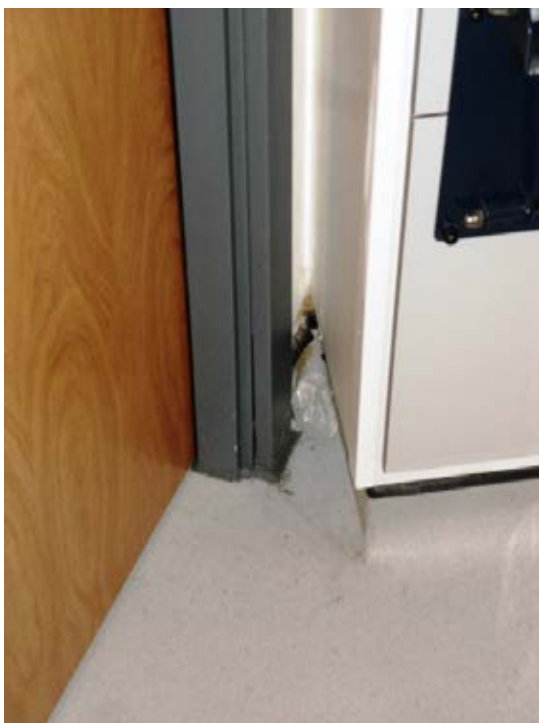
Poor vinyl detail at recess.
