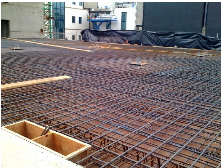
10. 3rd Floor Reinforcement at the Energy Centre.
