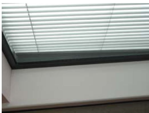
Blind not fitted in the window properly.
