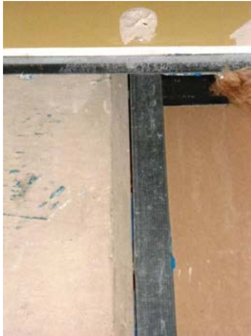
Insufficient seal between column and stud
