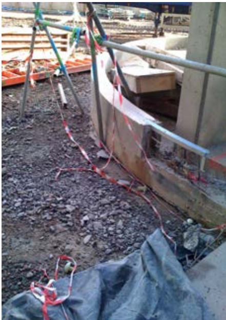
2 & 3. DPC Around Pod Floor Slab: 19 November 2010
