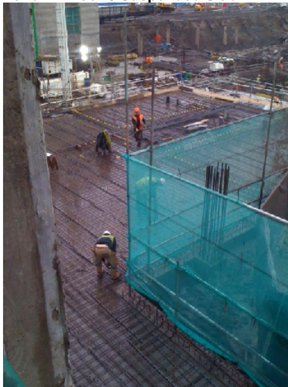
Zone E Floor 0 Suspended Slab
