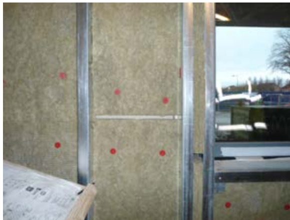
Gaps between insulation.
