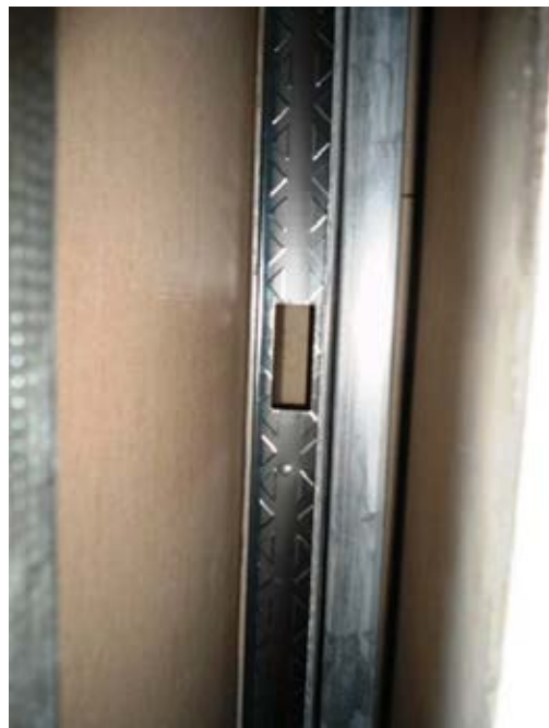
No insulation at end of partition
