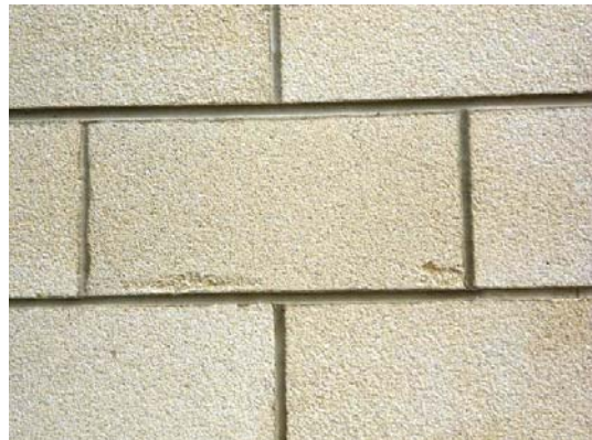
Damaged blockwork and overspill of mortar pointing at edge of blockwork.
