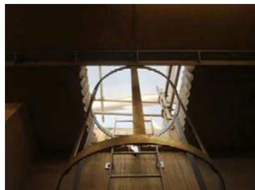
Hatch required to Cat ladder in room
