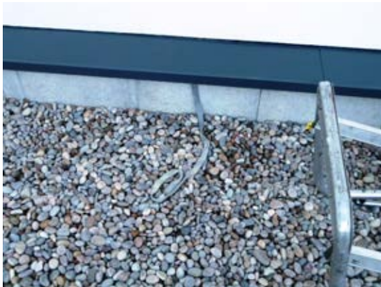
Lightning conductor tape not fitted.
