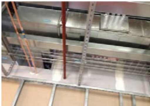
Example of new access hatch formed.
