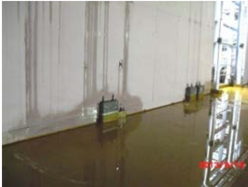
Water damaged boards.
