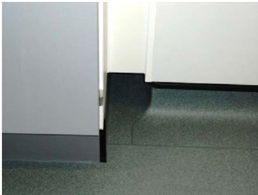
Gap between sink base unit and wall.
