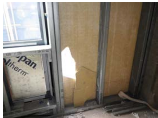
Damaged Board.
