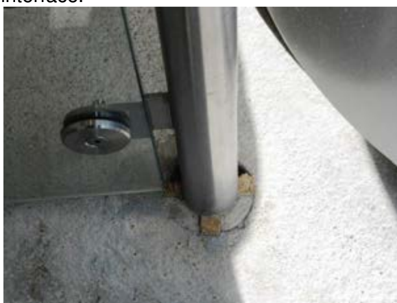
Timber wedges inappropriately used to support glazed panels.
