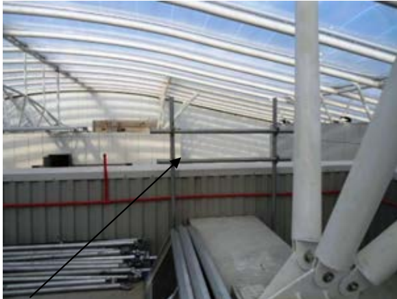
Temporary scaffolding providing perimeter protection.
