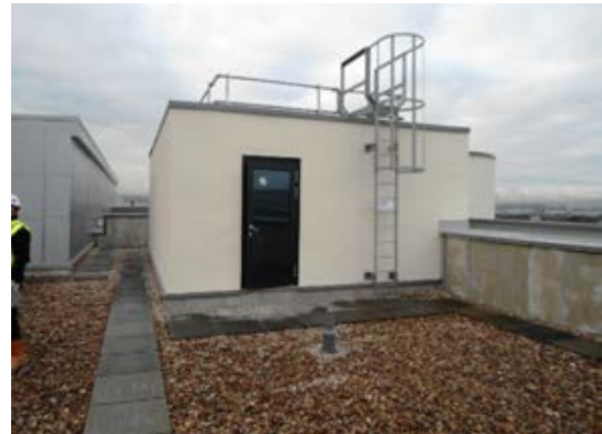
Access cat ladder should be fitted to this elevation.
