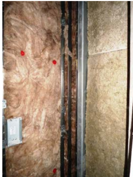
Junction of partition with external wall
