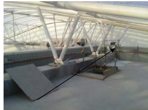
Temporary scaffolding providing perimeter protection.
