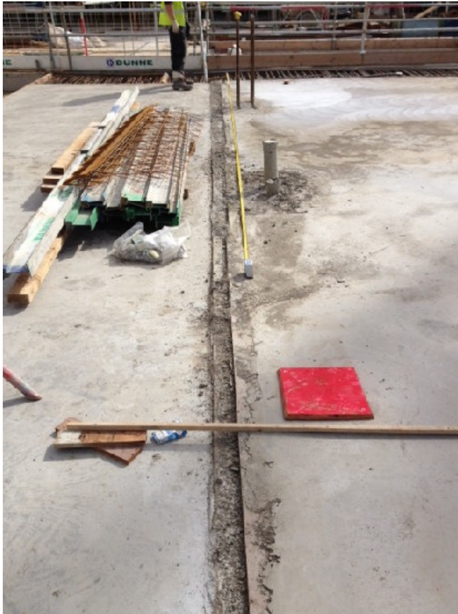
Photo 5 – change of level detail in 1st floor slab at Zone E
