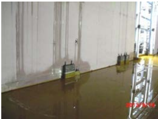
Water damaged boards.
