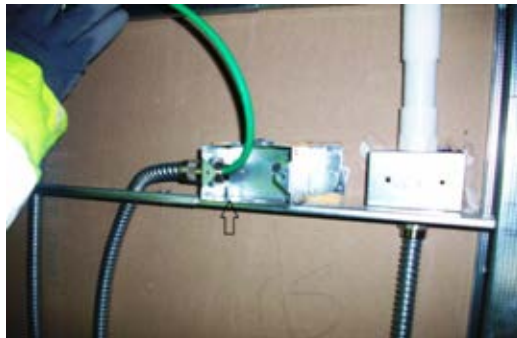
Screws fixed through back boxes.
