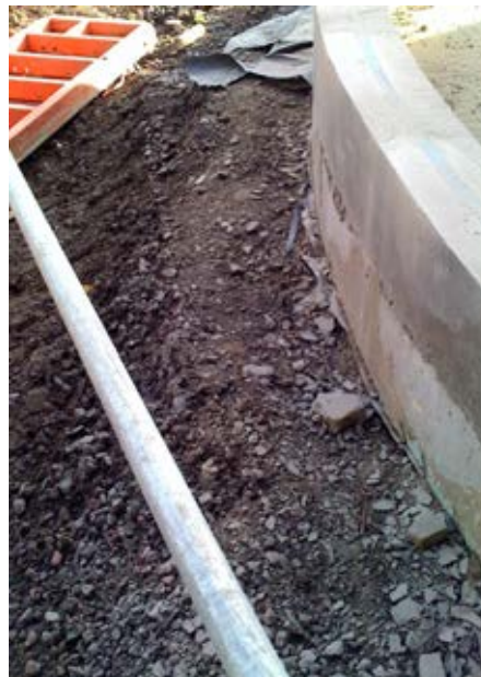
2 & 3. DPC Around Pod Floor Slab: 19 November 2010
