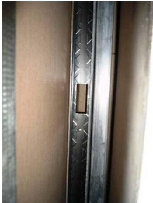
No insulation at end of partition
