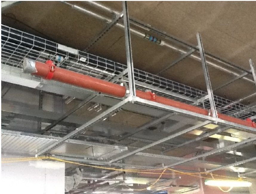
Photo No 3. Open ends of pipework sealed.
