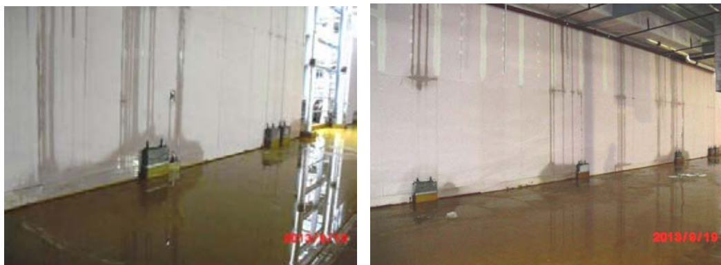
Water damaged boards.
