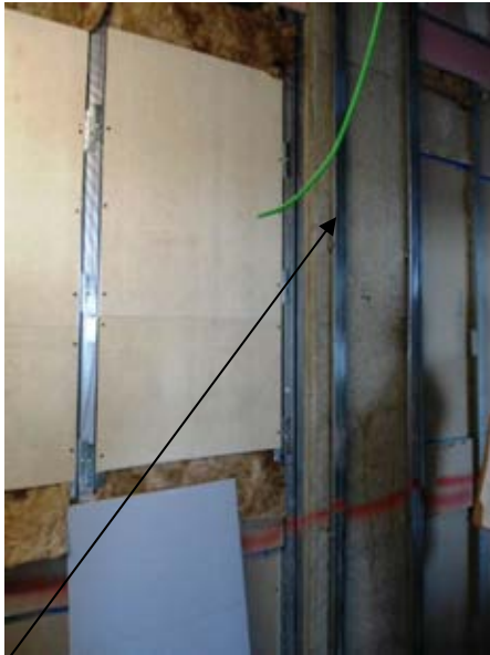
Double stud resulting failure of insulation qualities of partition.
