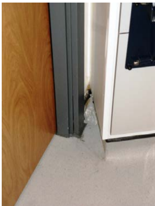
Poor vinyl detail at recess.
