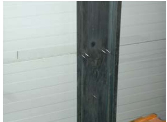
Unprotected screws.
