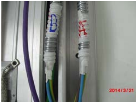
Metaflex cable incorrectly installed with PVC tape.
