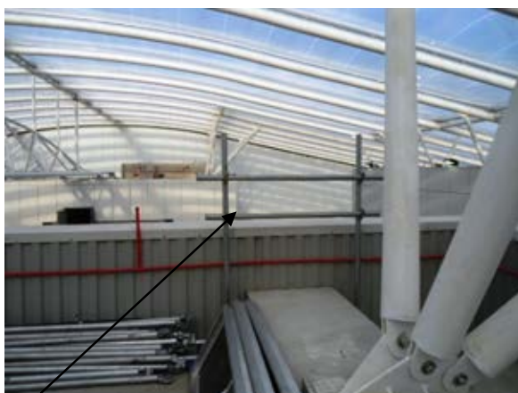
Temporary scaffolding providing perimeter protection.
