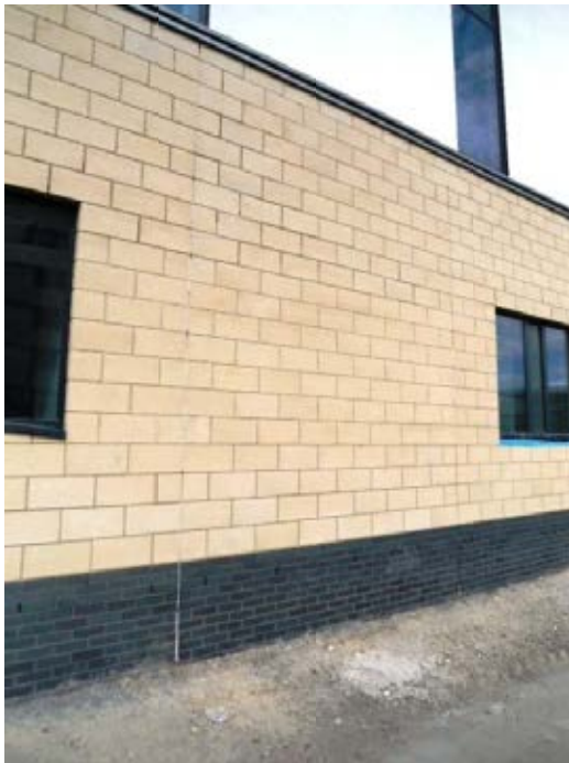
Shading of mortar pointing.
