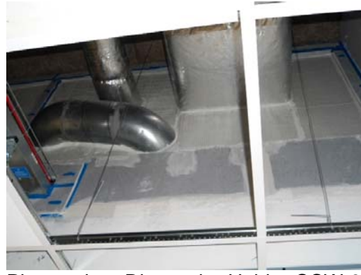
Photo in Disposal Hold CCW-034 showing ducting passing through in to Fluid Hold CCW-033.
