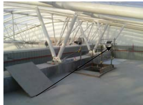
Temporary scaffolding providing perimeter protection.
