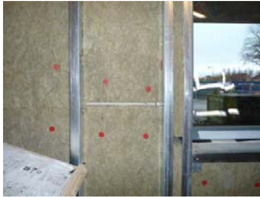
Gaps between insulation.
