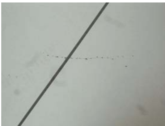
Two of the tiles has impact damage caused by what appears to be from an external source.
