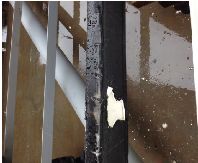
Photo 3 – Damaged intumescent cover.
