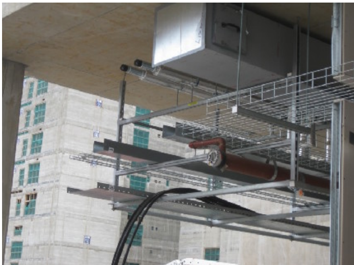
Photo 4 – M&E Installation Rig with Pipework Ends.
