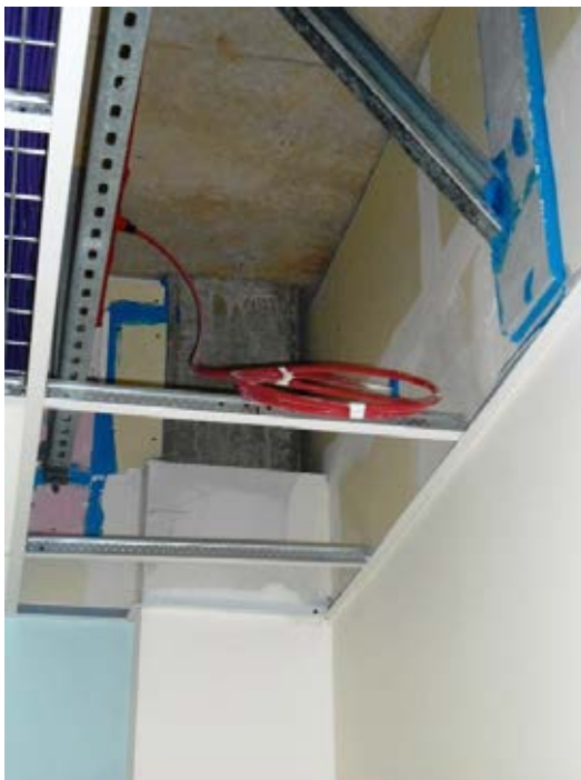
Opening between column and partition.
