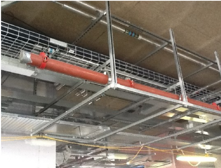
Photo No 3. Open ends of pipework sealed.
