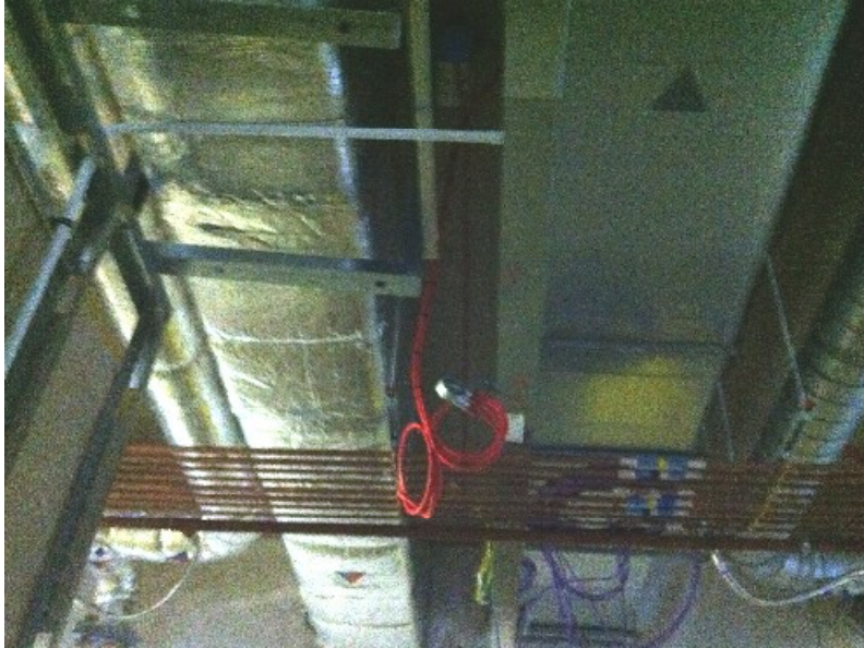
Photo 7 – ZG corridor CCW115 void detection has been located in close proximity and between ventilation ductwork.
