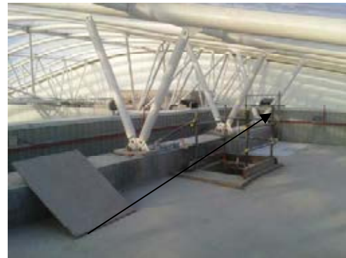
Temporary scaffolding providing perimeter protection.
