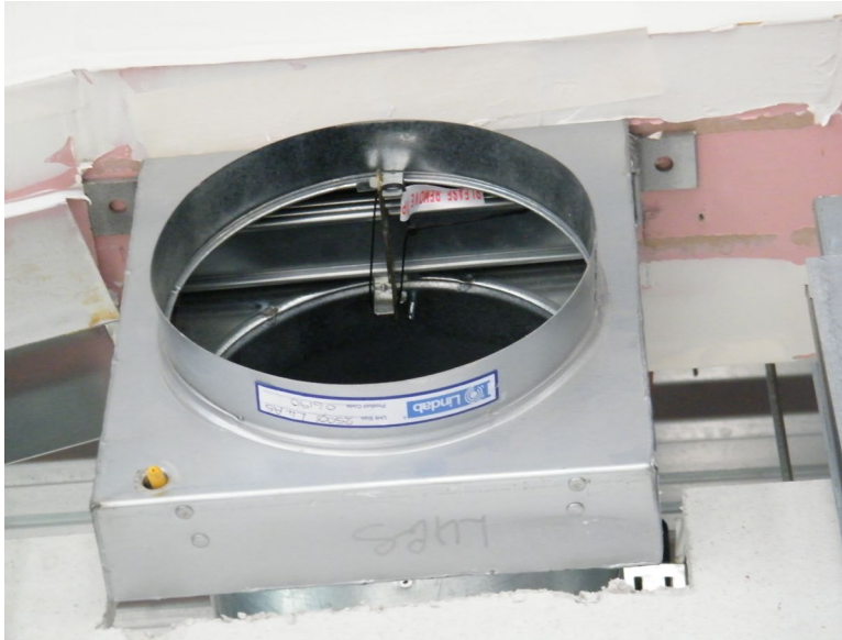
4. Fire Damper no fix to structure May 2011.
