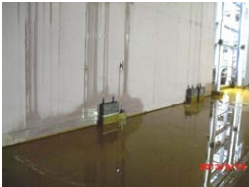
Water damaged boards.
