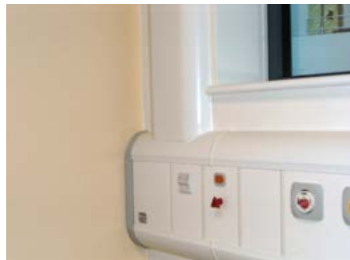
Bedhead junction at the horizontal vertical sections currently fitted on Level 1, Area 1-537 and 1-539 showing sealant.
