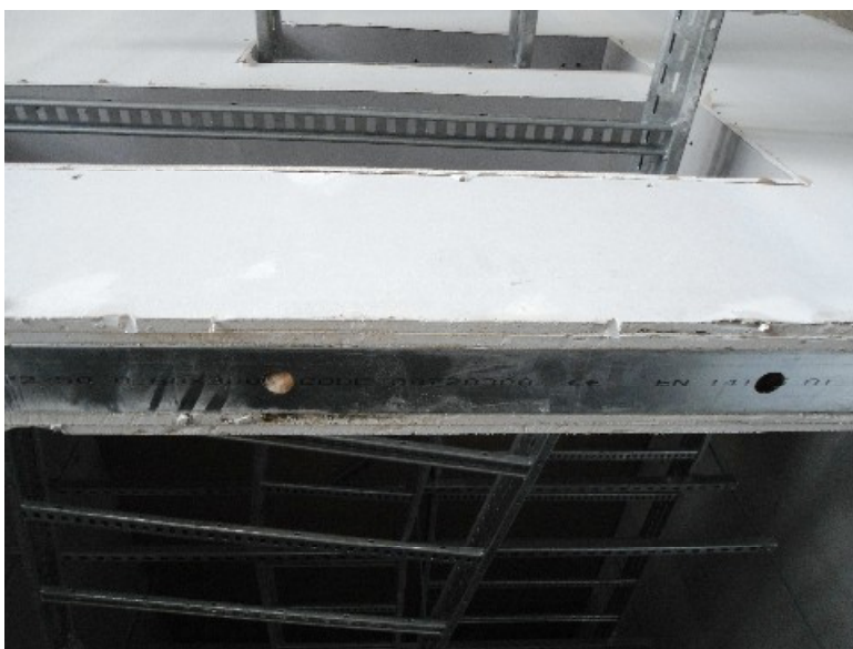
Photo 6 – Timber infill missing from lintel.
