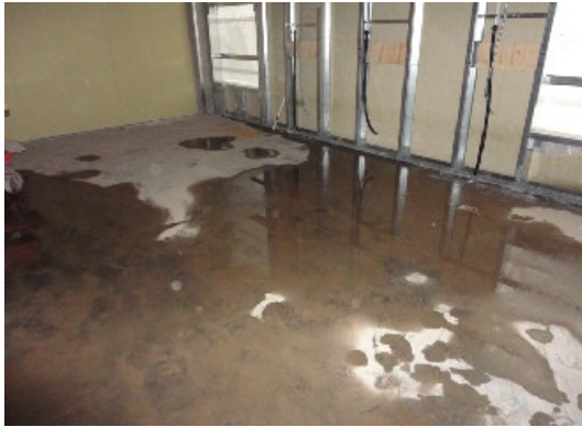
Water ingress as a result of rain penetration through wall.
