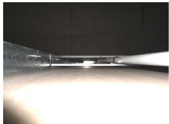
No insulation at high level.
