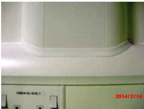
Bedhead junction at the horizontal vertical sections currently fitted on Level 0 showing gasket.
