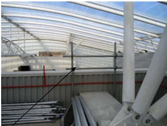
Temporary scaffolding providing perimeter protection.
