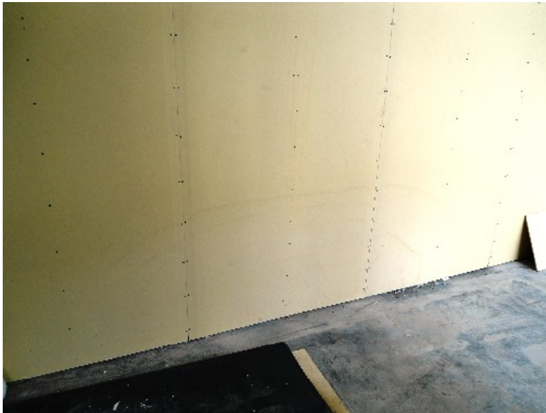
Photo 3 – Water stained boards Core E Stair Lobby Level 2
