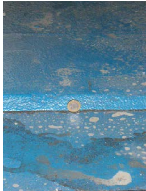
Level 3: Channel exceeds 30mm deep.
