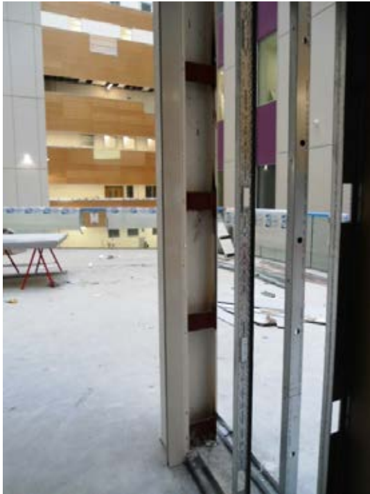
Steel cleats without intumescent paint.
