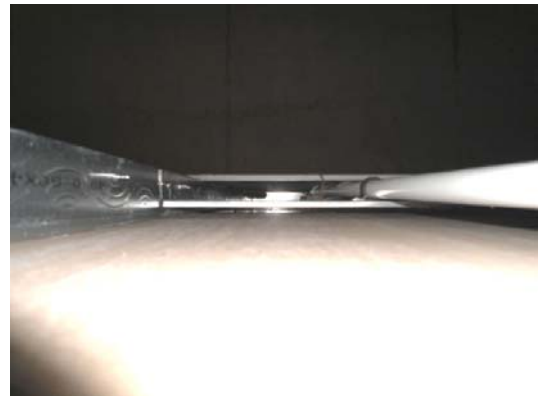
No insulation at high level.
