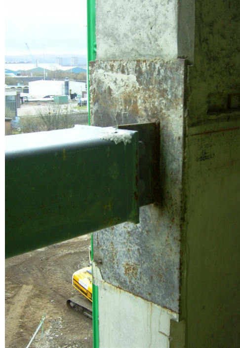
2. Rust on steel plate April 2011.
