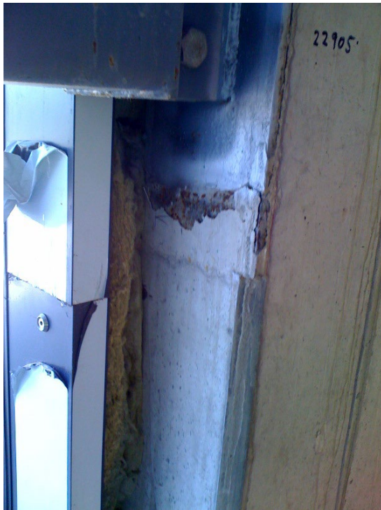
10. Incomplete touch up painting to the steel plates at the stairwells April 2011.
