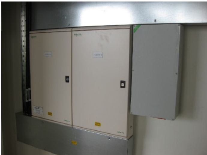
Photo 2 – Distribution Boards installed, Cables Terminated
