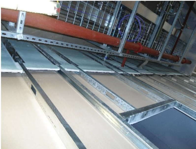
Photo 5 – Insulation not fitted to shaftwall.
