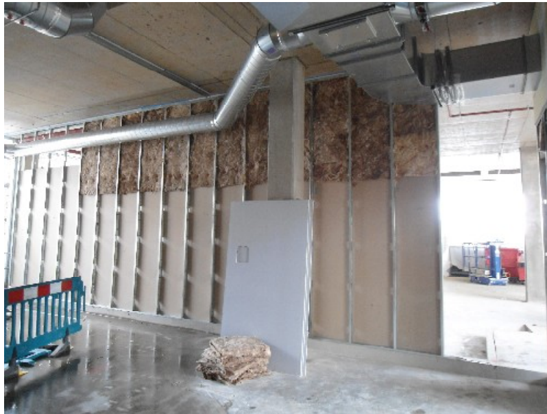
Photo 7 – Room THE-171 no insulation.
