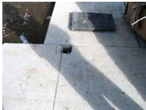
Damaged insulation
