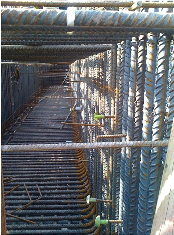
Reinforcing Core C
