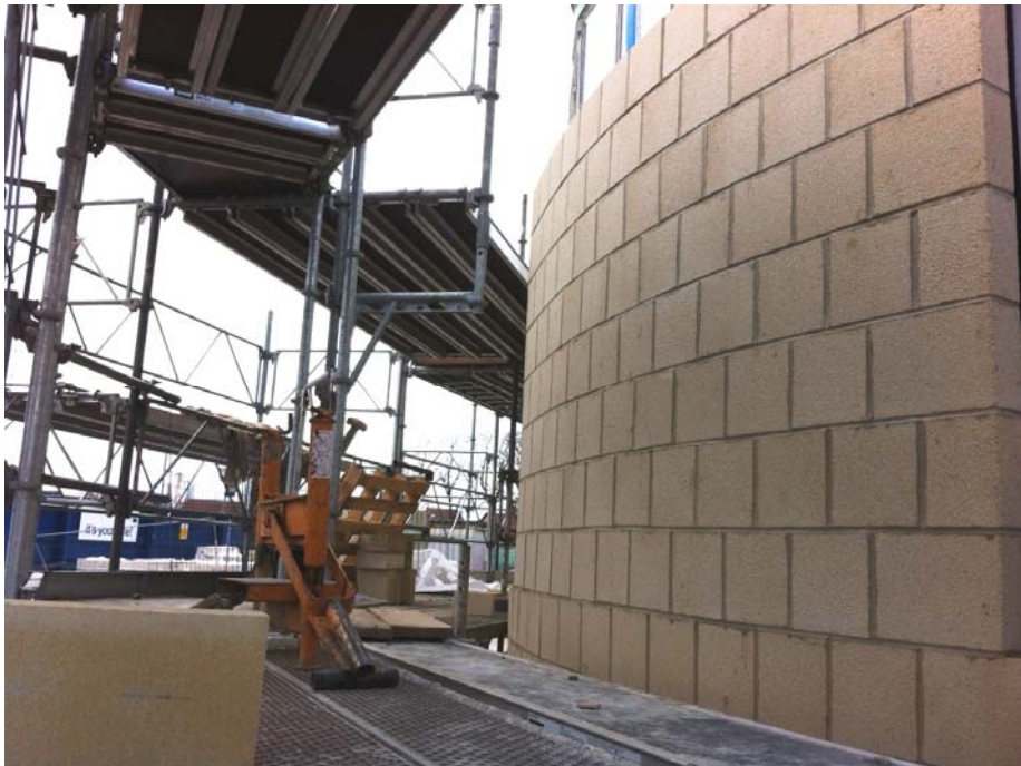
Poor quality blockwork with irregular beds and poor pointing
