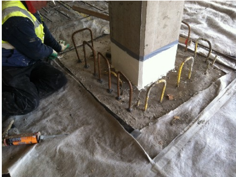
Photo 4 – New U bars drilled in 200 deep with resin anchor fixing.
