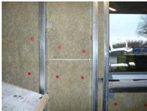
Gaps between insulation.
