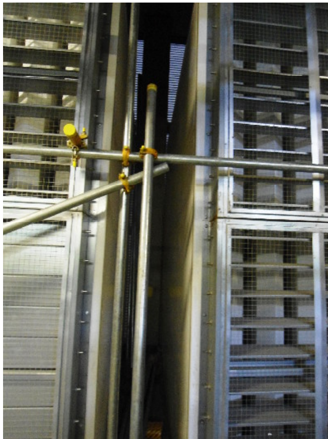
Photo 8 – Gap between acoustic intake louvers.
