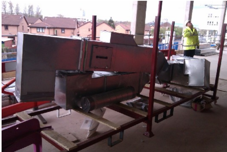
Photo No 5. Ductwork Delivery Method
