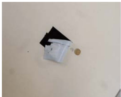
Tile in the Children's Hospital located opposite room CCO-047 has impact damage caused by what appears to be from an external source.
