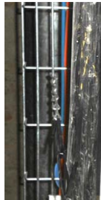
Restricted access to smoke detector.
