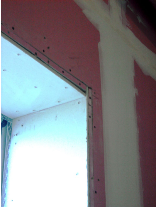
1. Poor plasterboard detail Level 1 West Elevation.
