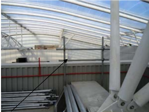
Temporary scaffolding providing perimeter protection.
