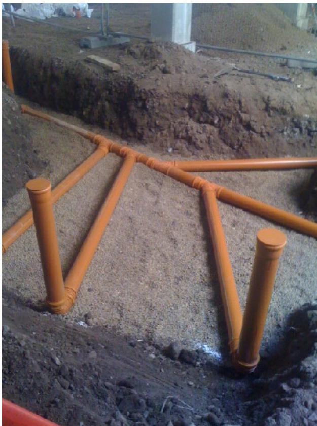
Photo No 4. Drainage installation.
