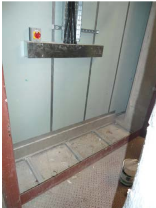
Gap between the metal deck and the wall with the floor comprising fire bats.
