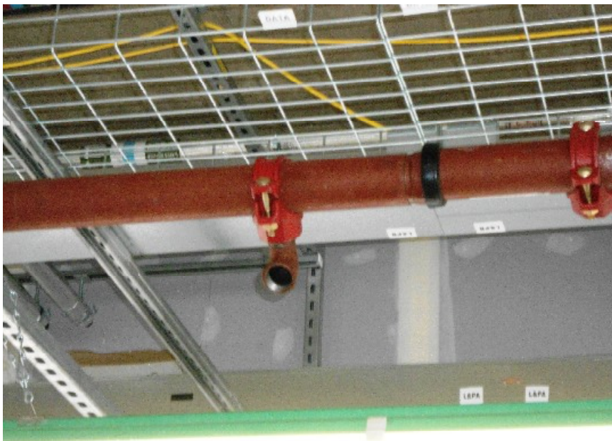
Photo No 2. Open ends of pipework
