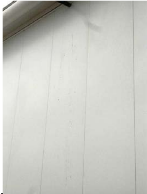
Pigeon droppings on cladding of Core B
