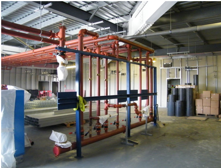
5. Pump / pipework support not fixed at top May 2011.
