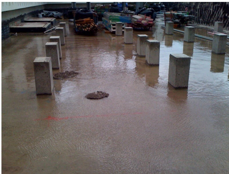
3. Ponding due to roof not laid to falls May 2011.
