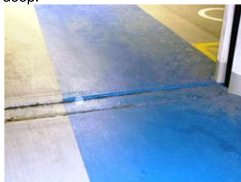
Level 3: Channel exceeds 30mm deep.
