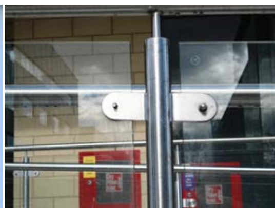
Nuts not fitted to glazed fixings to ramp.
