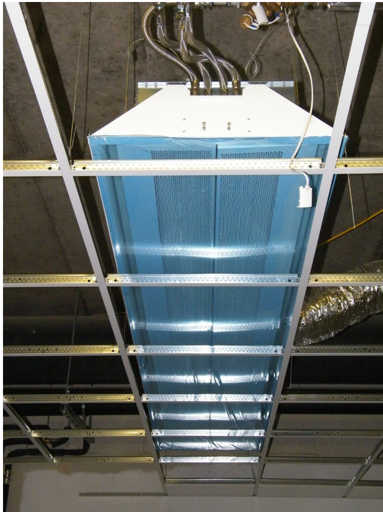
8. Chilled Beams not aligned and supports not suitable May 2011.
