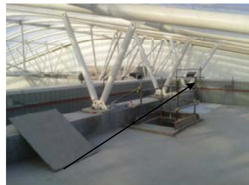
Temporary scaffolding providing perimeter protection.
