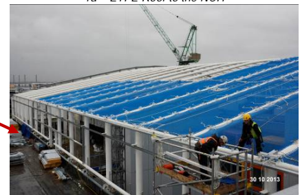
1b - Installation of netting and ETFE - adult atrium roof
