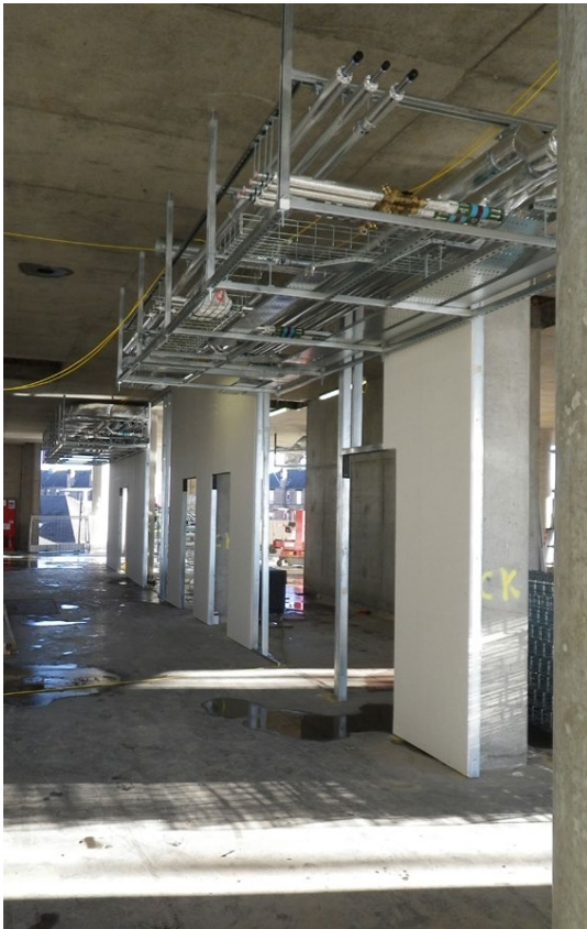
Internal fit out – a service pod in place
