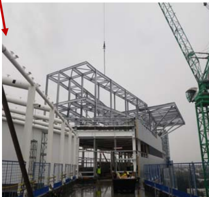
1d – Helipad steelwork
