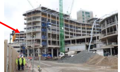
Hoists installed so materials can be delivered into the building
