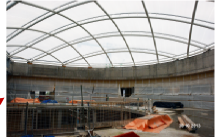
1a – ETFE Roof to the NCH
