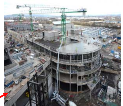
Plantroom steelwork being erected and concrete slab being poured
