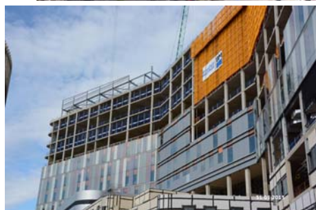
1c - Curtain walling to the east elevation
