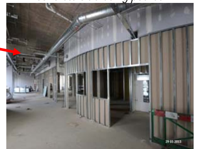
Partitions being installed to NCH general ward area (level 3)
