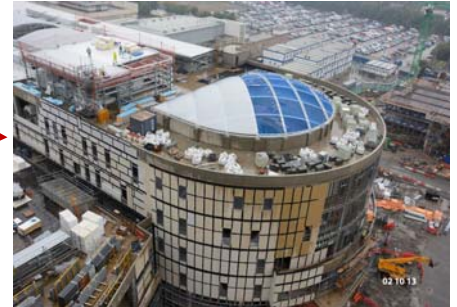
1a – ETFE Roof being installed to the NCH
