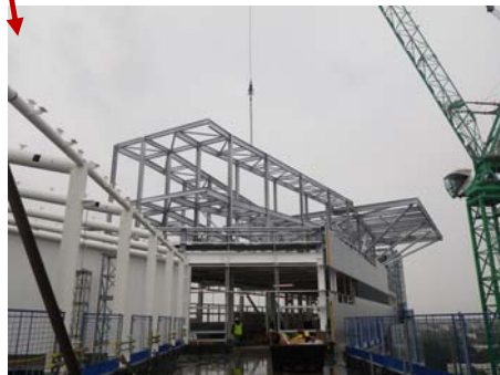
1d – Helipad steelwork
