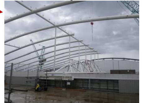
1b - Installation of the steel for the adult atrium roof
